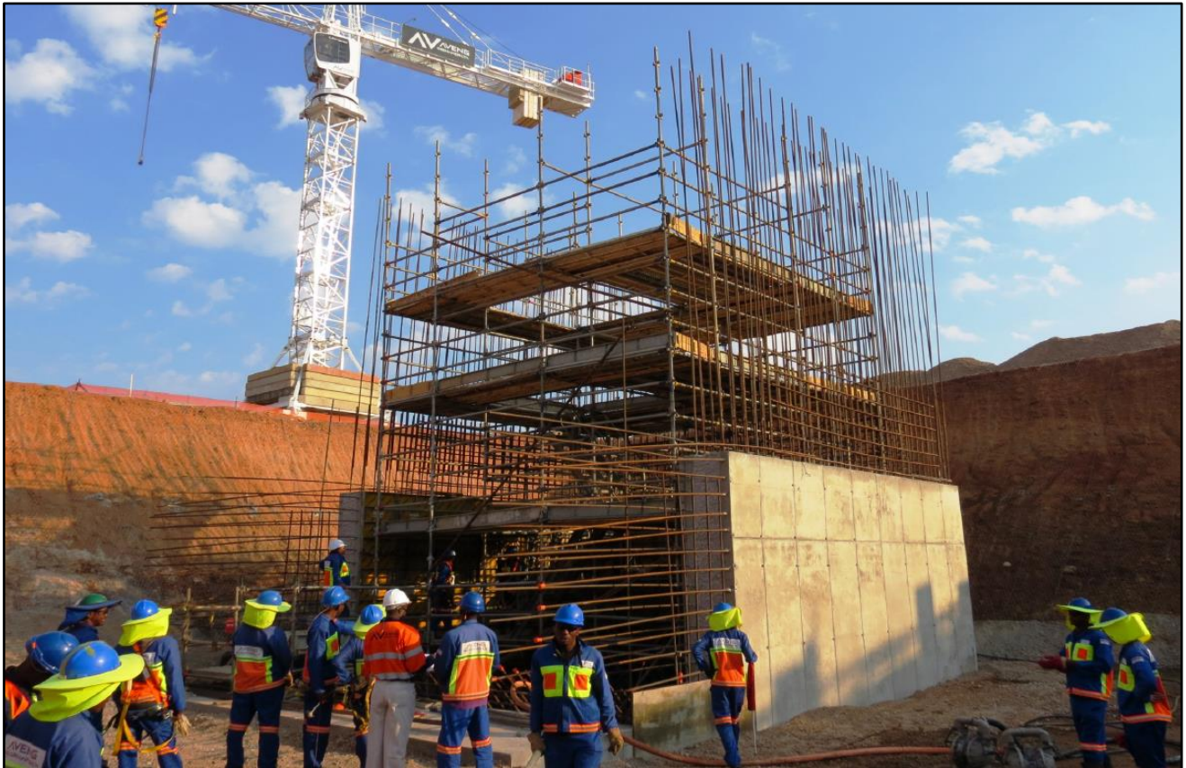
Figure 5: Construction of Shaft 1 collar, May 8, 2015.
