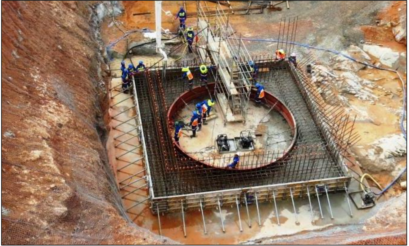
Figure 5: Construction of Shaft 1 collar, May 8, 2015.
