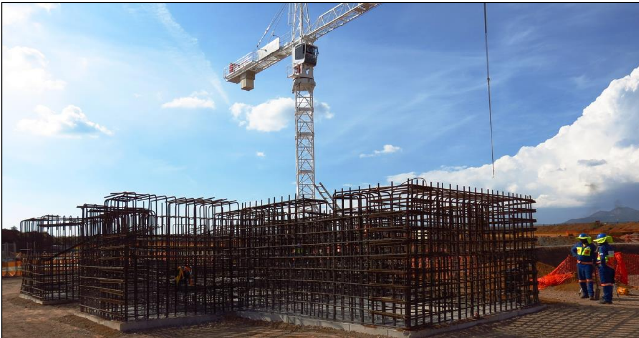
Figure 6: Construction of Shaft 1 kibble winder foundation.
