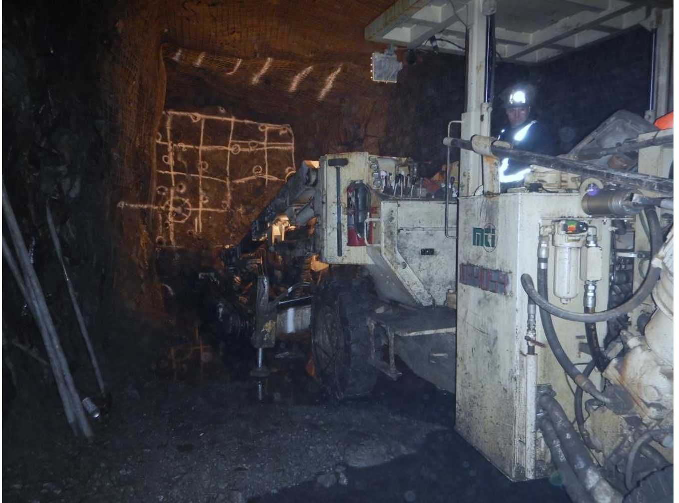
Figure 4: Underground development at Trevali's Caribou Mine
