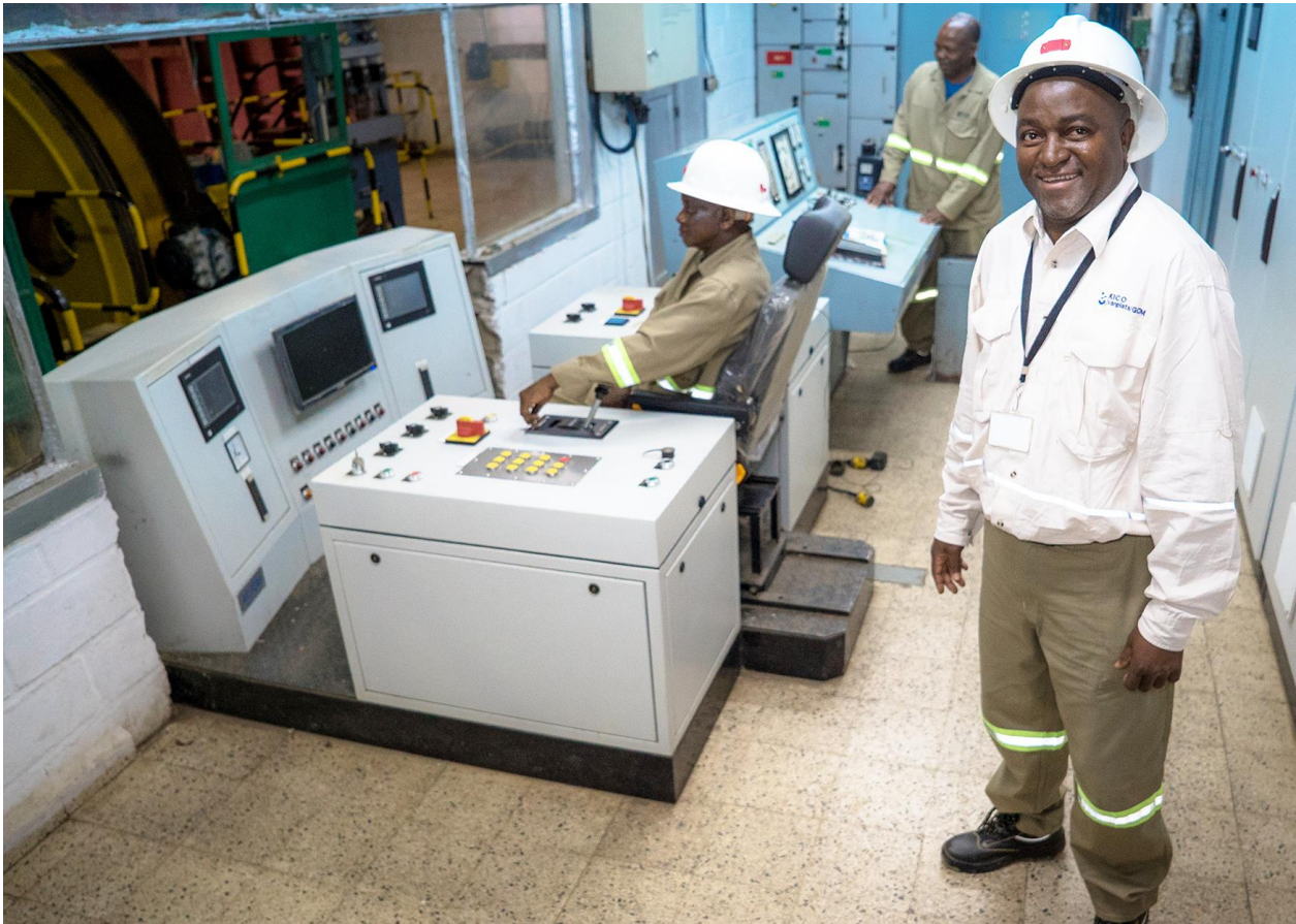
Figure 11: New winder control centre at Shaft 5.
