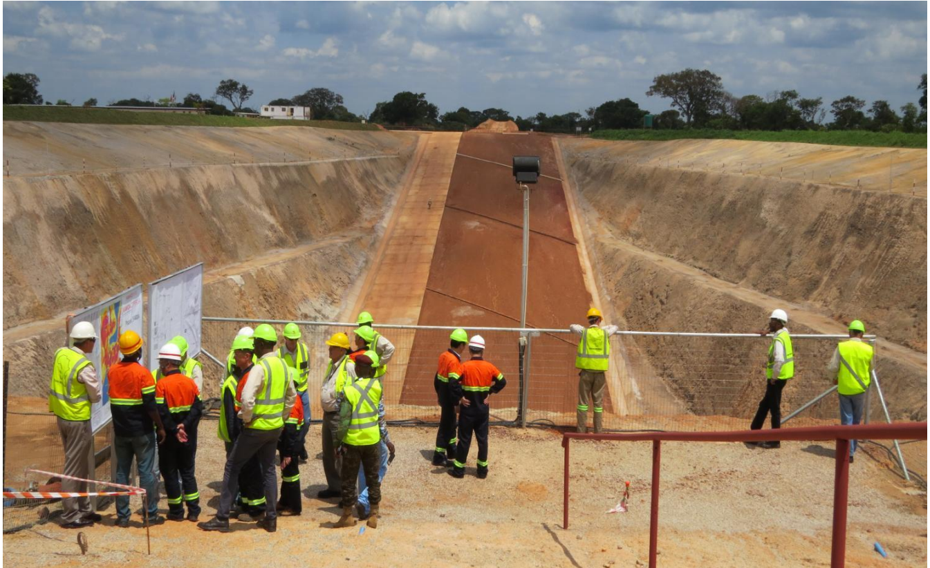
Box cut (portal) at Kamo'a's initial high-grade mining area — Kansoko Sud
