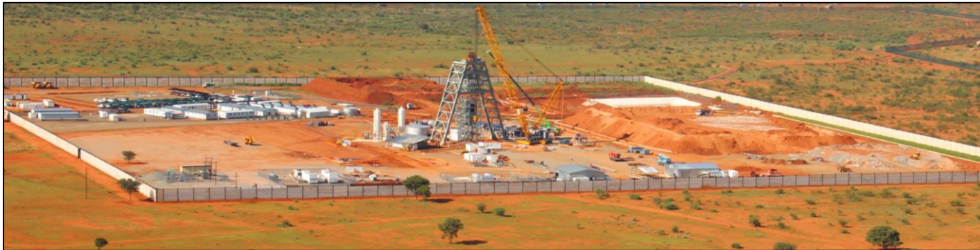
Figure 1: Aerial view of the Platreef Project site.
