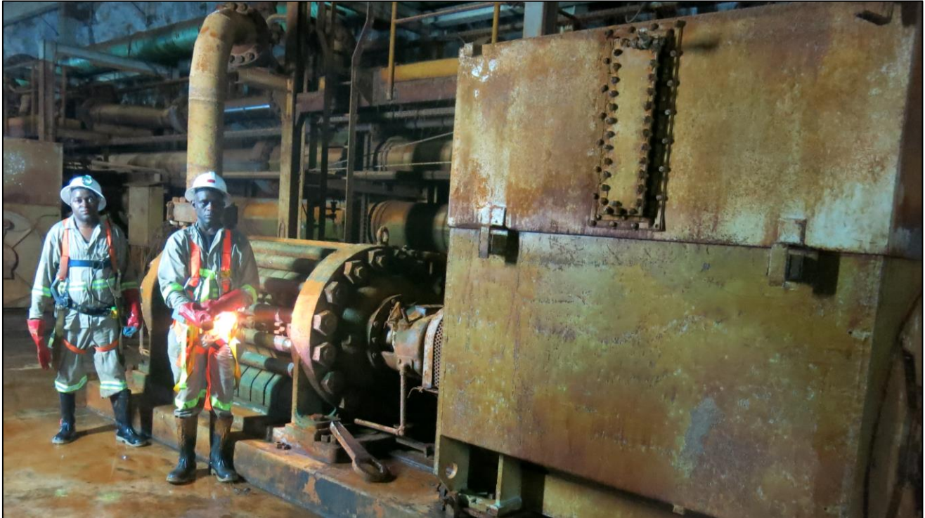
Figure 10: Sulzer centrifugal pump at the 1,200-metre-level pump station in Shaft 5.
