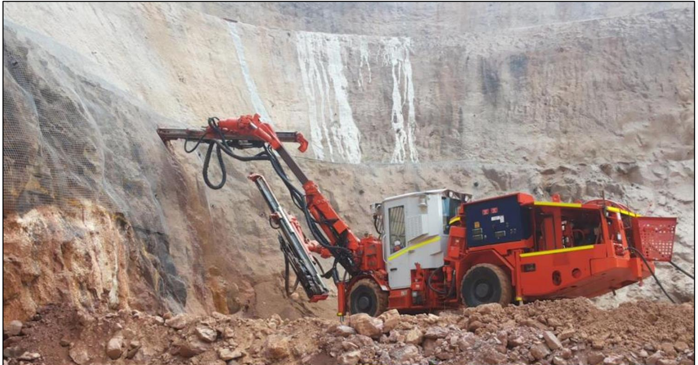
Figure 16: Drilling of anchor-bolt holes at the Kamo'a box cut.
