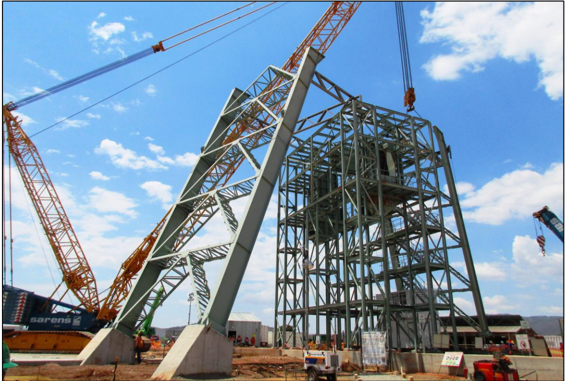
Figure 3: Construction of headgear for main sinking operations.
