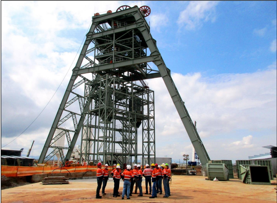
Figure 4: Shaft 1 main-sink headgear.
