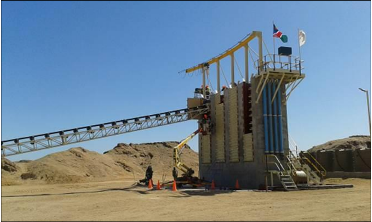
Figure 1 - Etango Heap Leach Demonstration Plant
