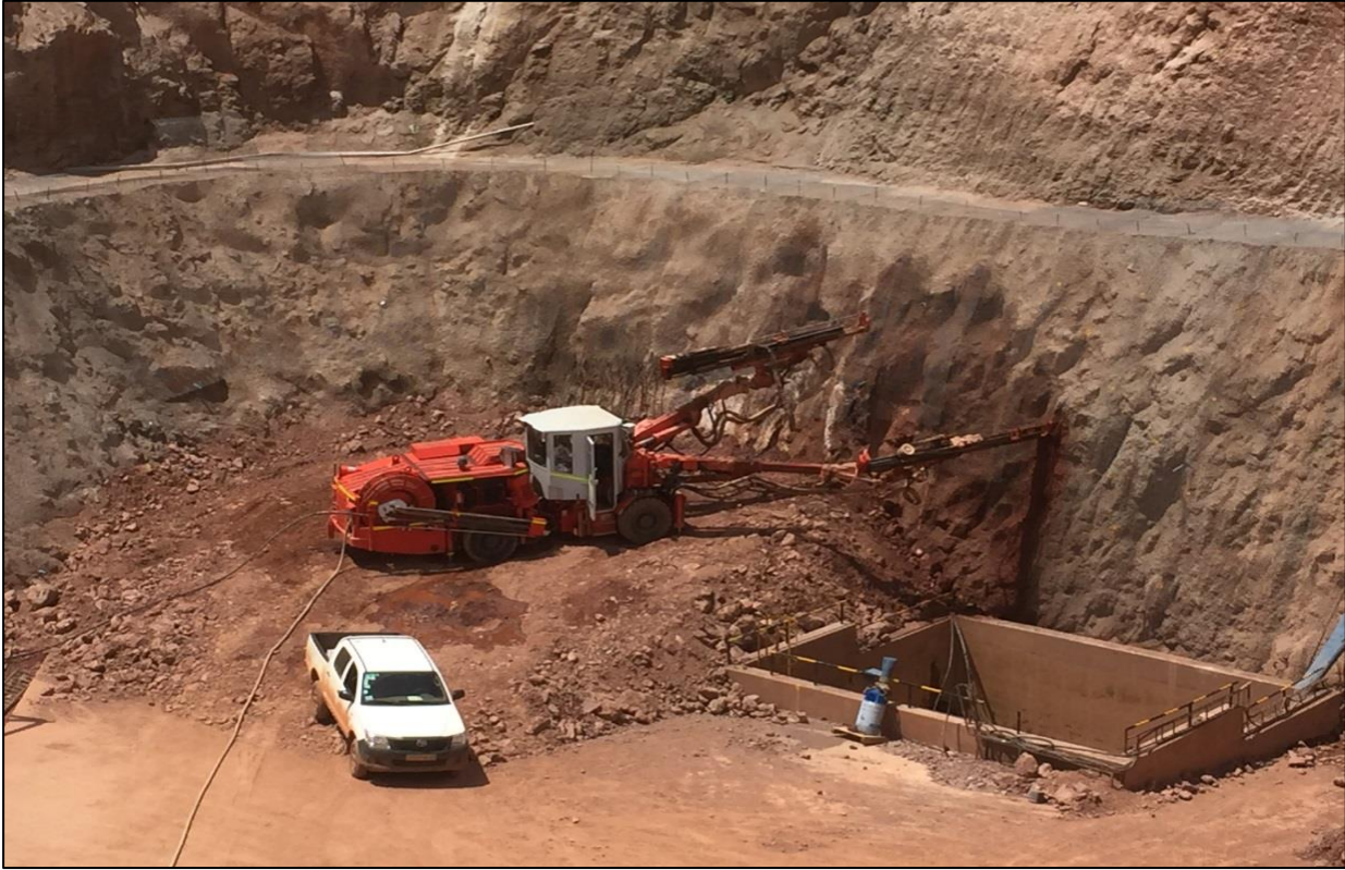
Double-boom drill rig drilling three-metre rebar holes on the bottom bench.
