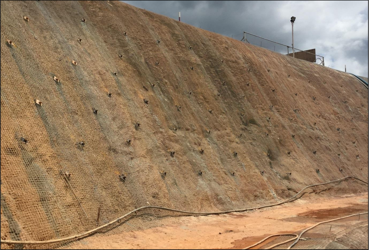
Installed mesh and three-metre rebar bolts.
