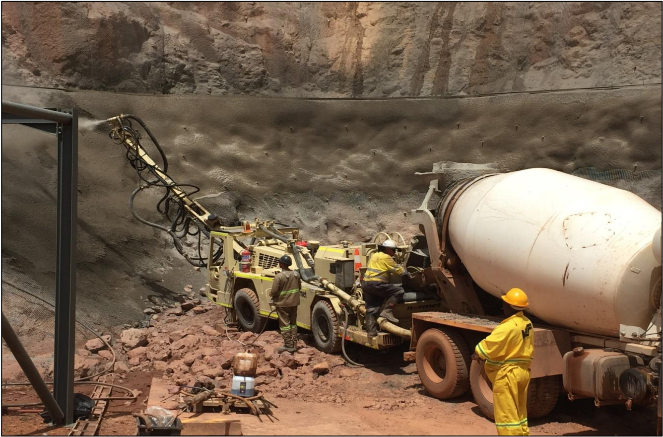
Shotcrete application on the bottom bench.
