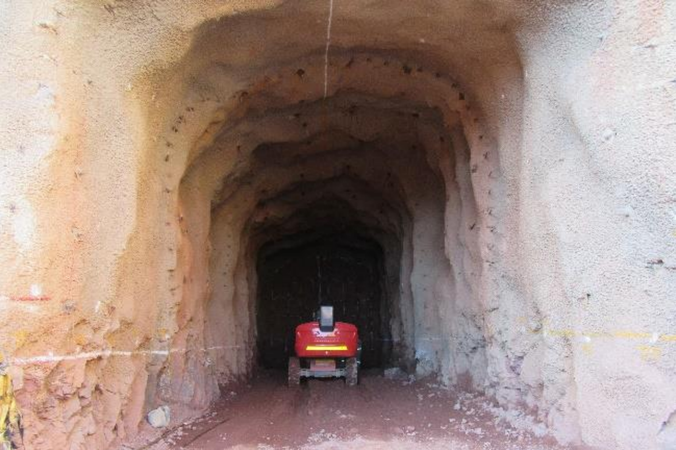
Preparations underway for another excavation blast in the service decline.
