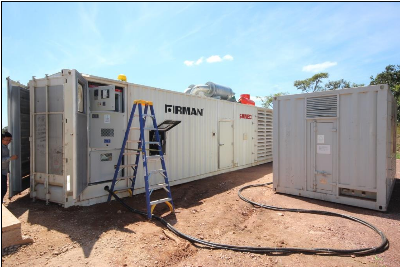
Figure 10. Sumec 2-MW generator being commissioned.
