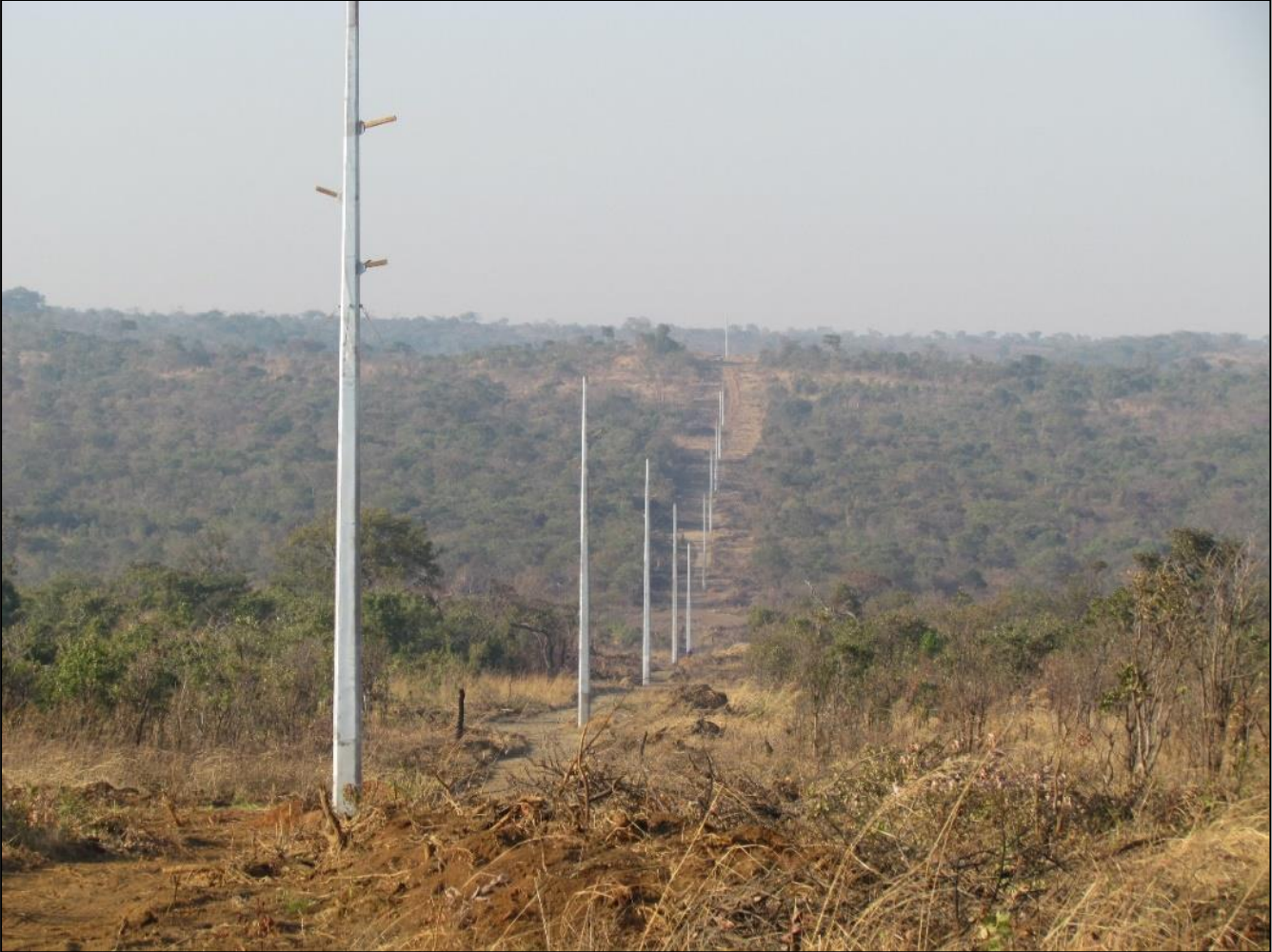
Figure 11. 120 kV power line under construction.
