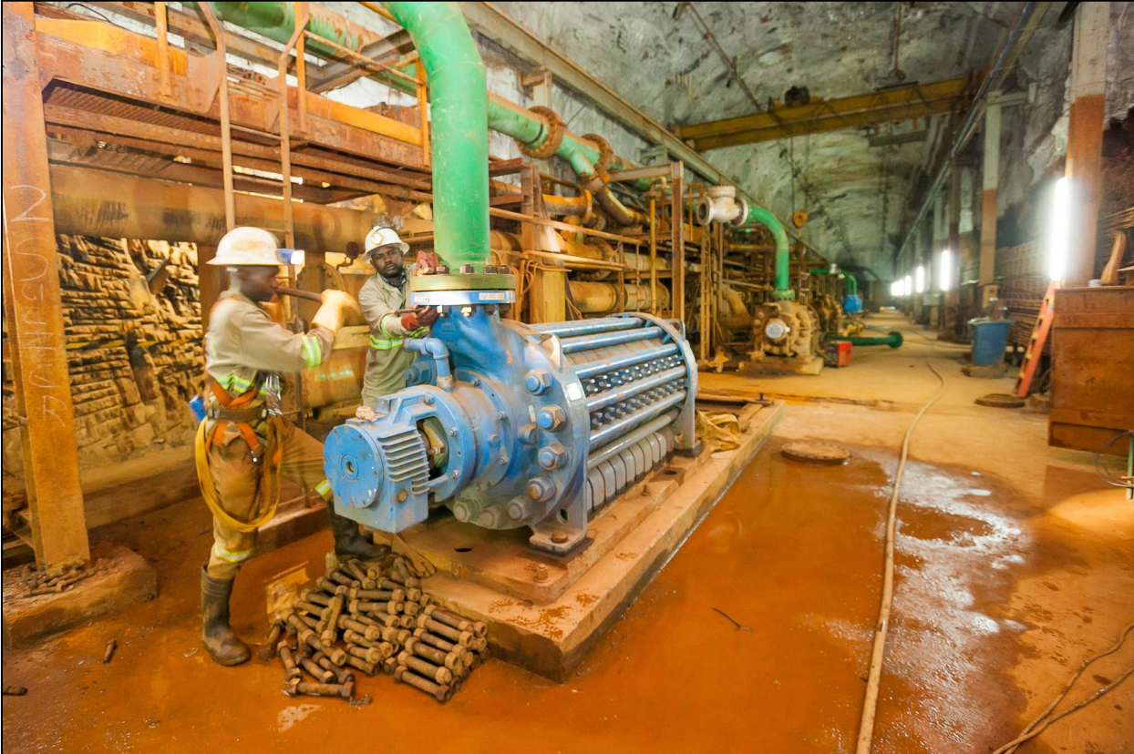
Figure 2. Main pump station in Shaft 5 at 1,200-metre-level with installation of Grifo centrifugal pump.
