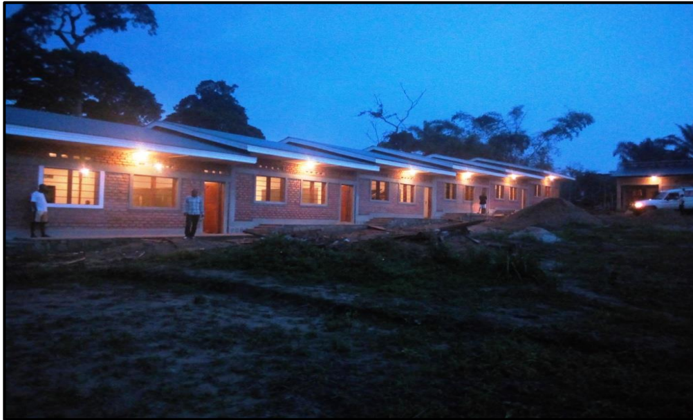
Figure 5: New School constructed at Logu
