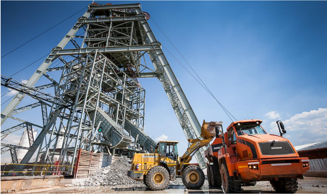
Figure 1. Platreef Project's Shaft 1 head gear, showing removal of excavated rock from shaft-sinking operations.
