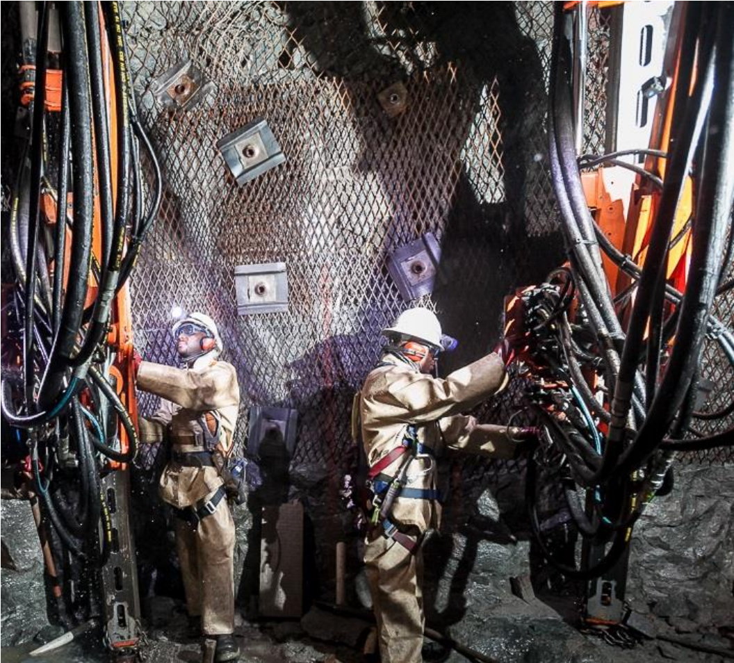
Figure 2. Shaft-sinking crew operating jumbo drill rigs underground in Shaft 1.
