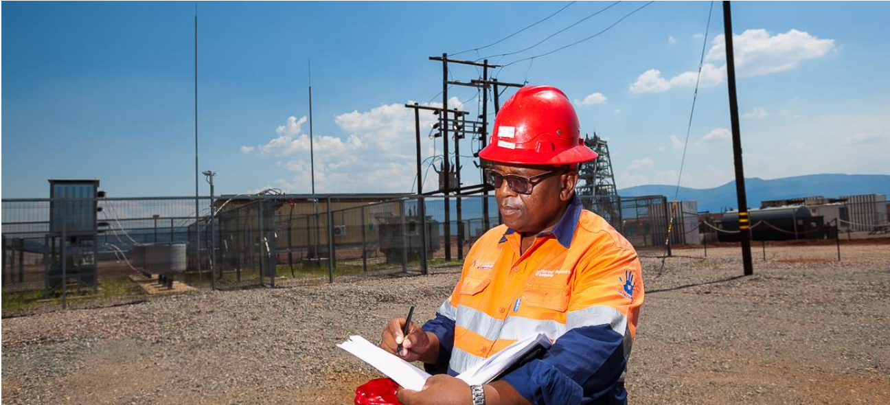
Figure 3. Eskom's five-million-volt-ampere power line, energized last month, now is supplying electricity from the national grid for shaft sinking and construction activities at Platreef.
