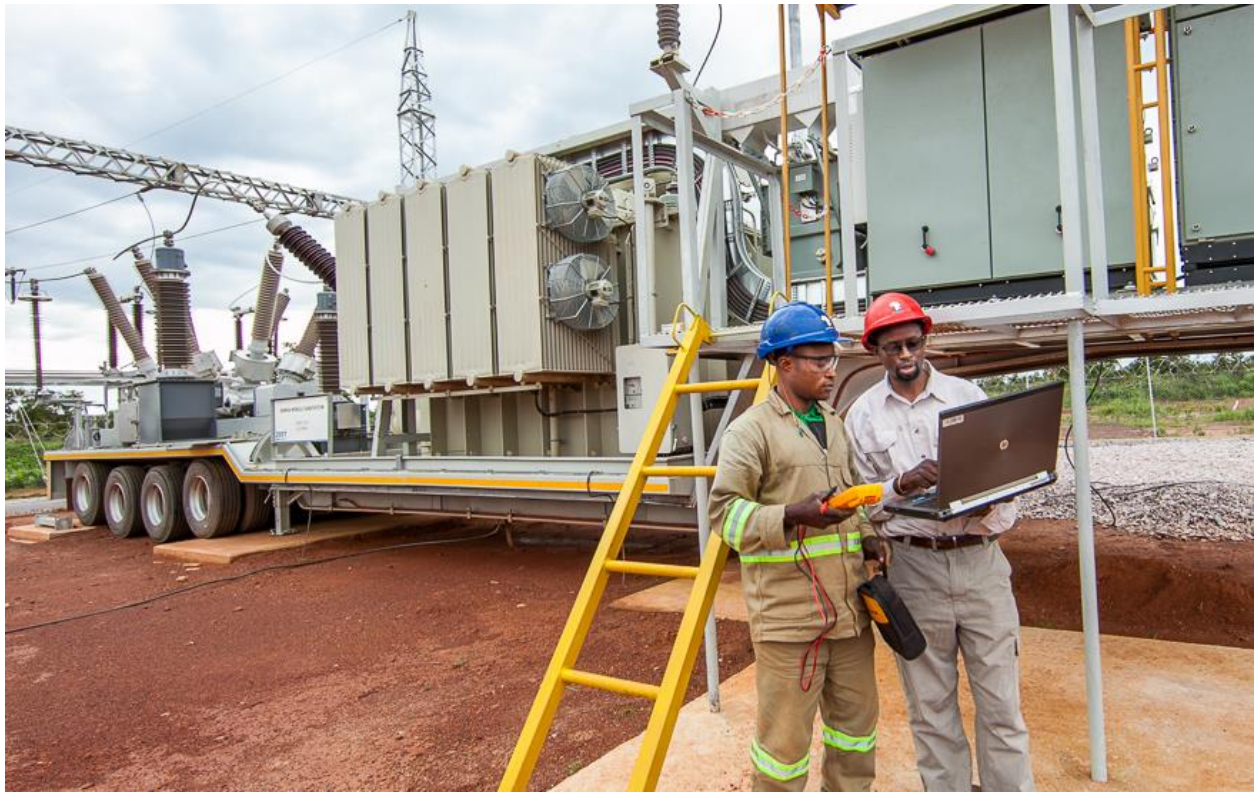
Figure 9: Kamoia-Kakula Project team members working on the 11-kilovolt mobile substation that is connected to the DRC national electricity grid now supplying power to develop the access declines for the planned mine.
