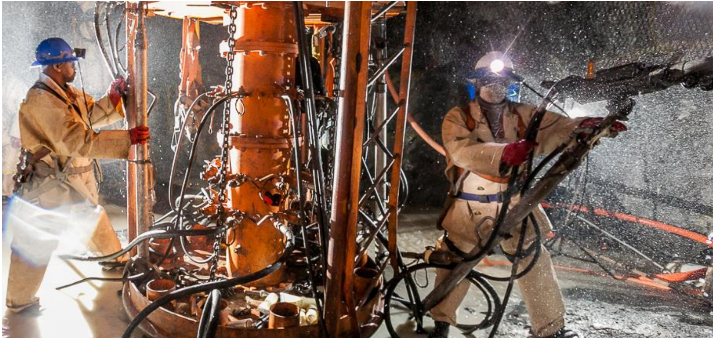
Shaft-sinking team members operating the jumbo drill in Shaft 1.
