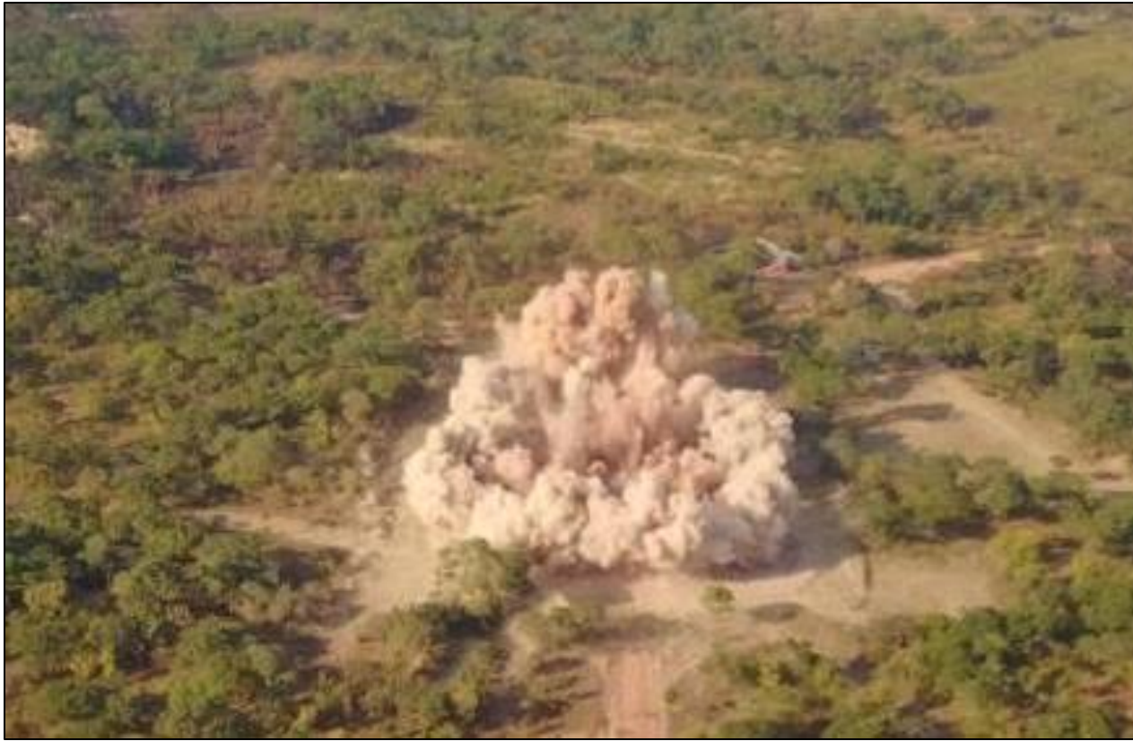
Figures 11 and 12: The first blast, followed by ongoing excavation work at the Kakula box cut.
