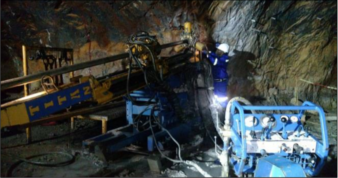
Figure 4: Kipushi underground drilling with one of Titan's drill rigs.
