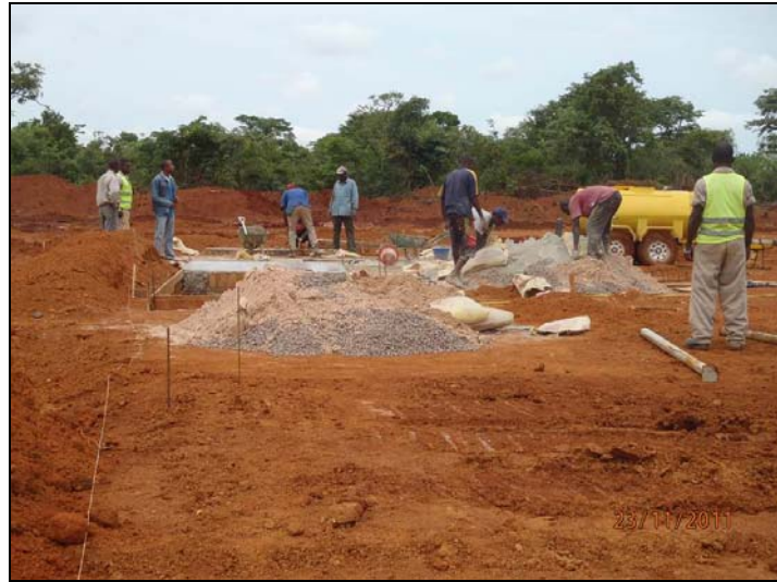
Photo 2: Sub-contract concreting team.
