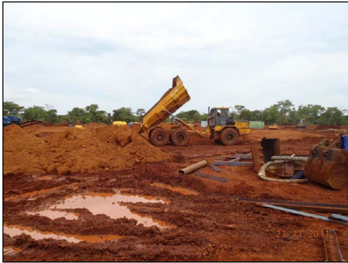
Photo 4: On-going site drainage works
