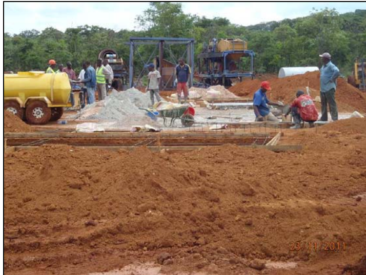
Photo 3: Sub-contract concreting team.
