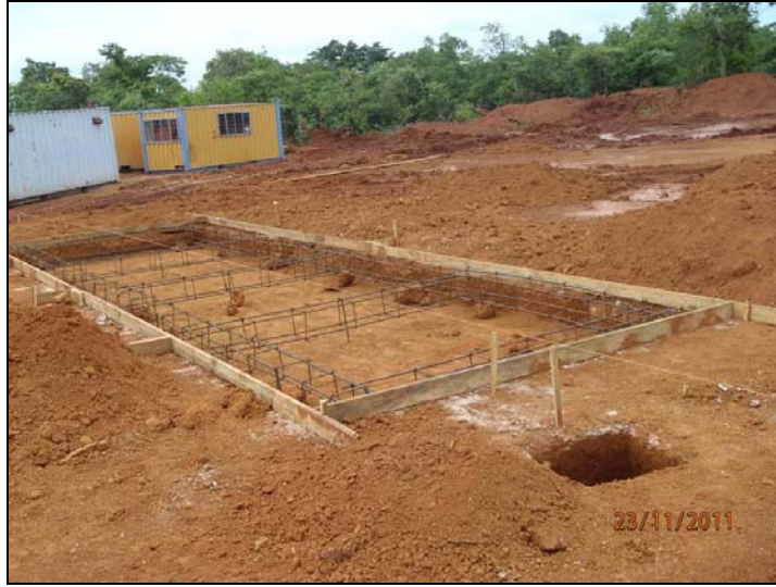
Photo 1: Boxing and preparation works for concrete footings.
