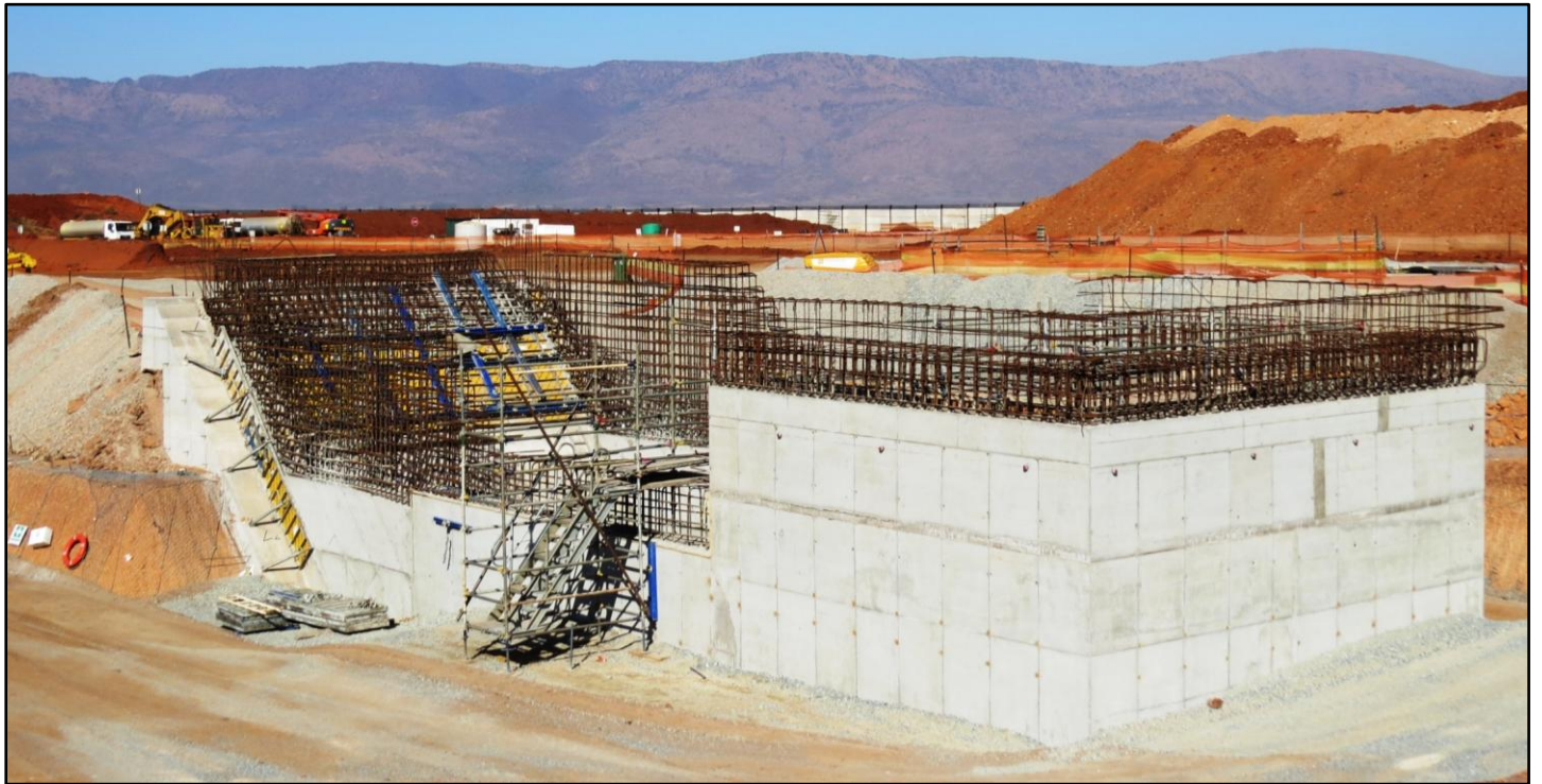
Figure 3: Shaft 1 collar and ventilation plenum construction, July 2015.
