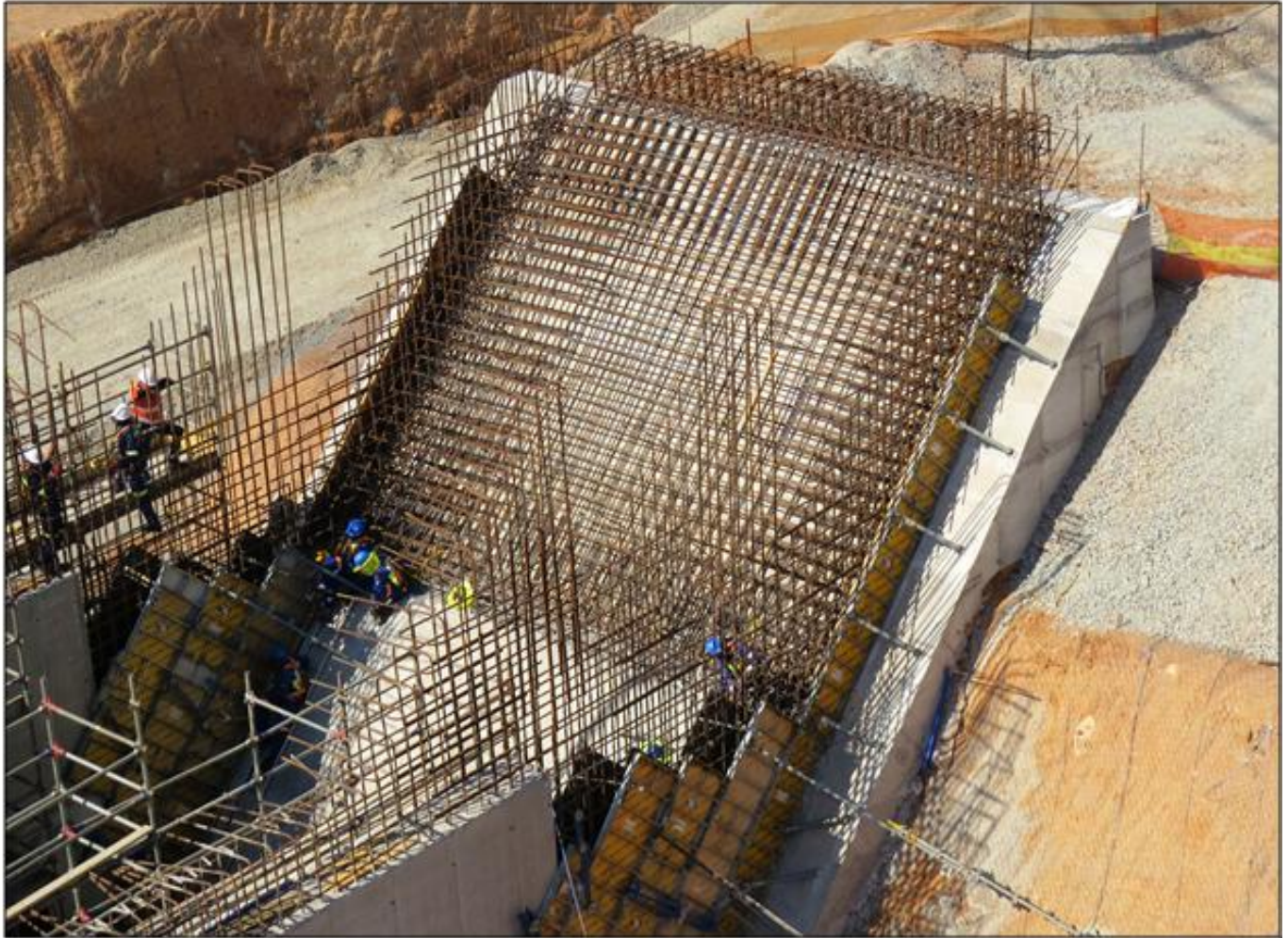
Figure 6: Construction of Shaft 1 ventilation plenum.
