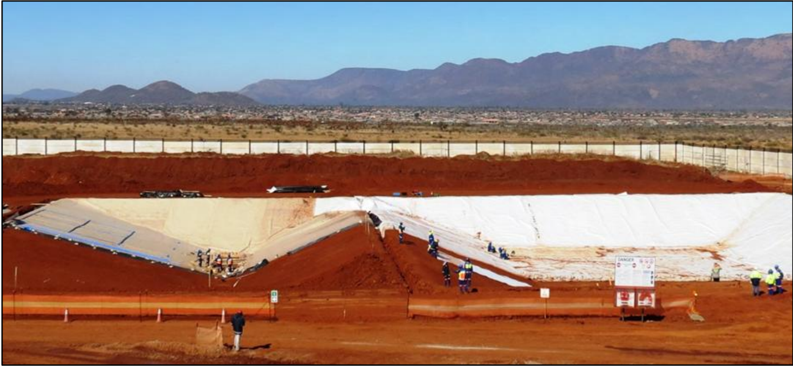
Figure 7: Construction of the lined storm-water pond.
