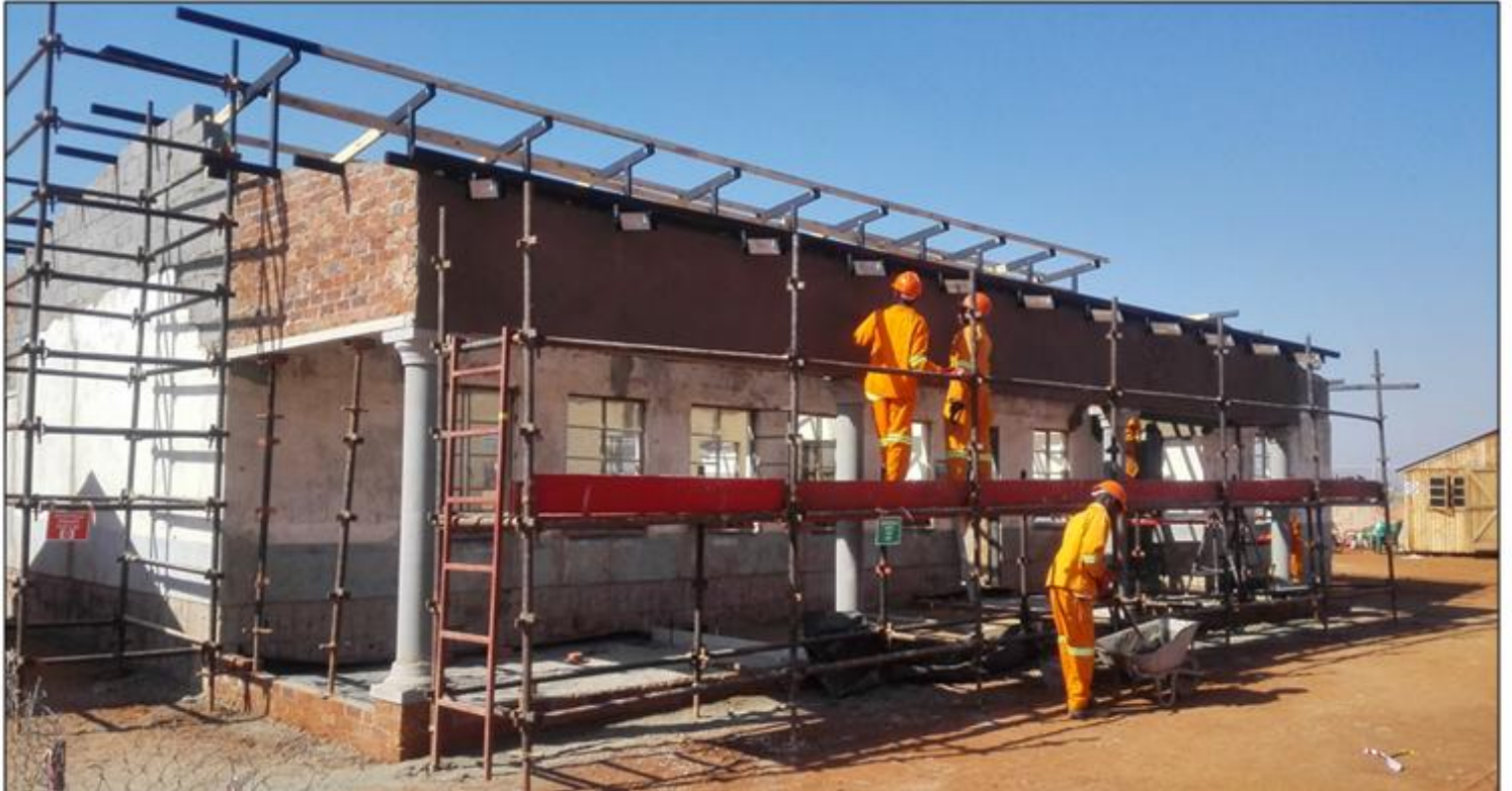
Figure 8: Renovation of a community care centre in a host village.
