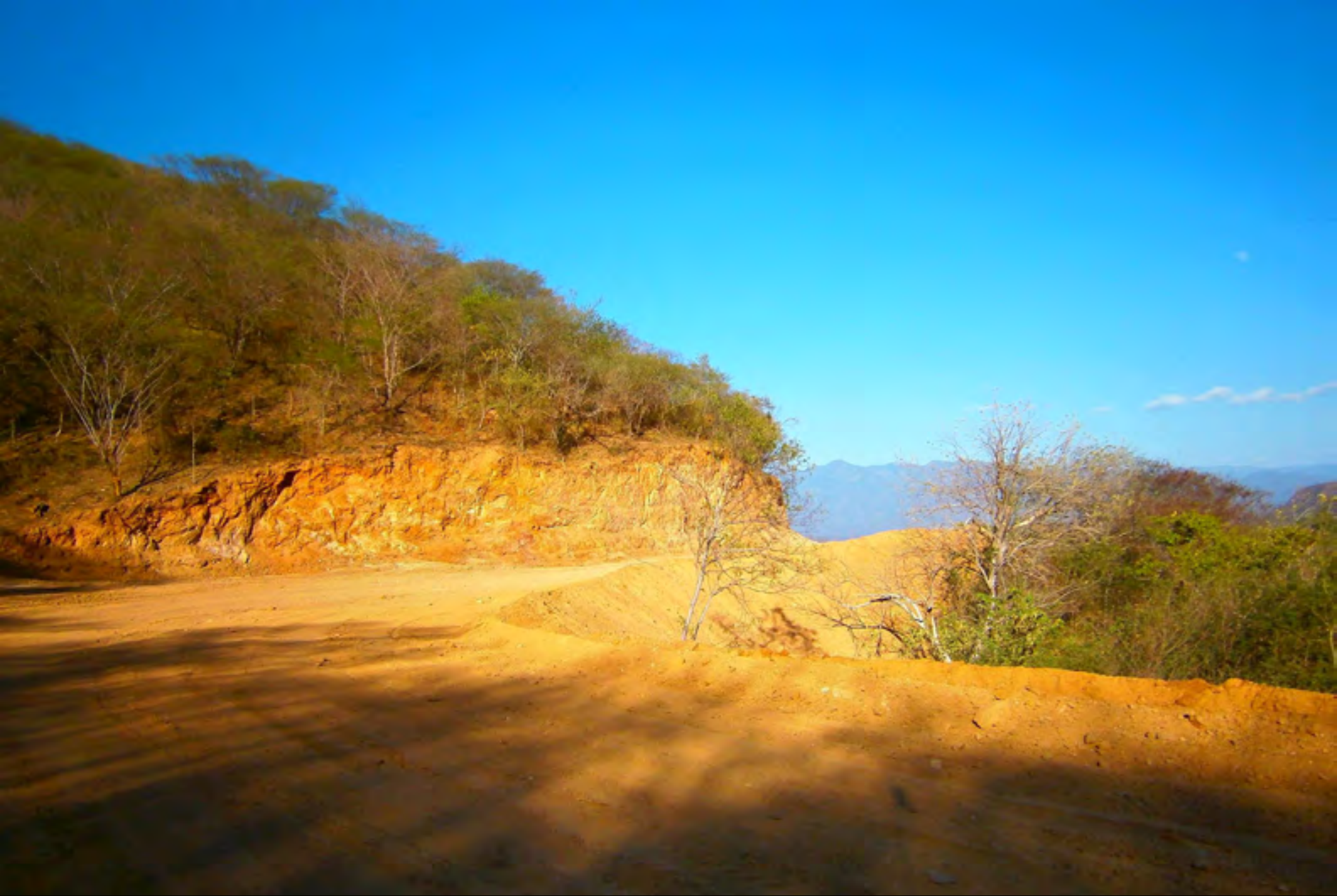
Haul road to the Sargrado Corzon deposit nears completion.
