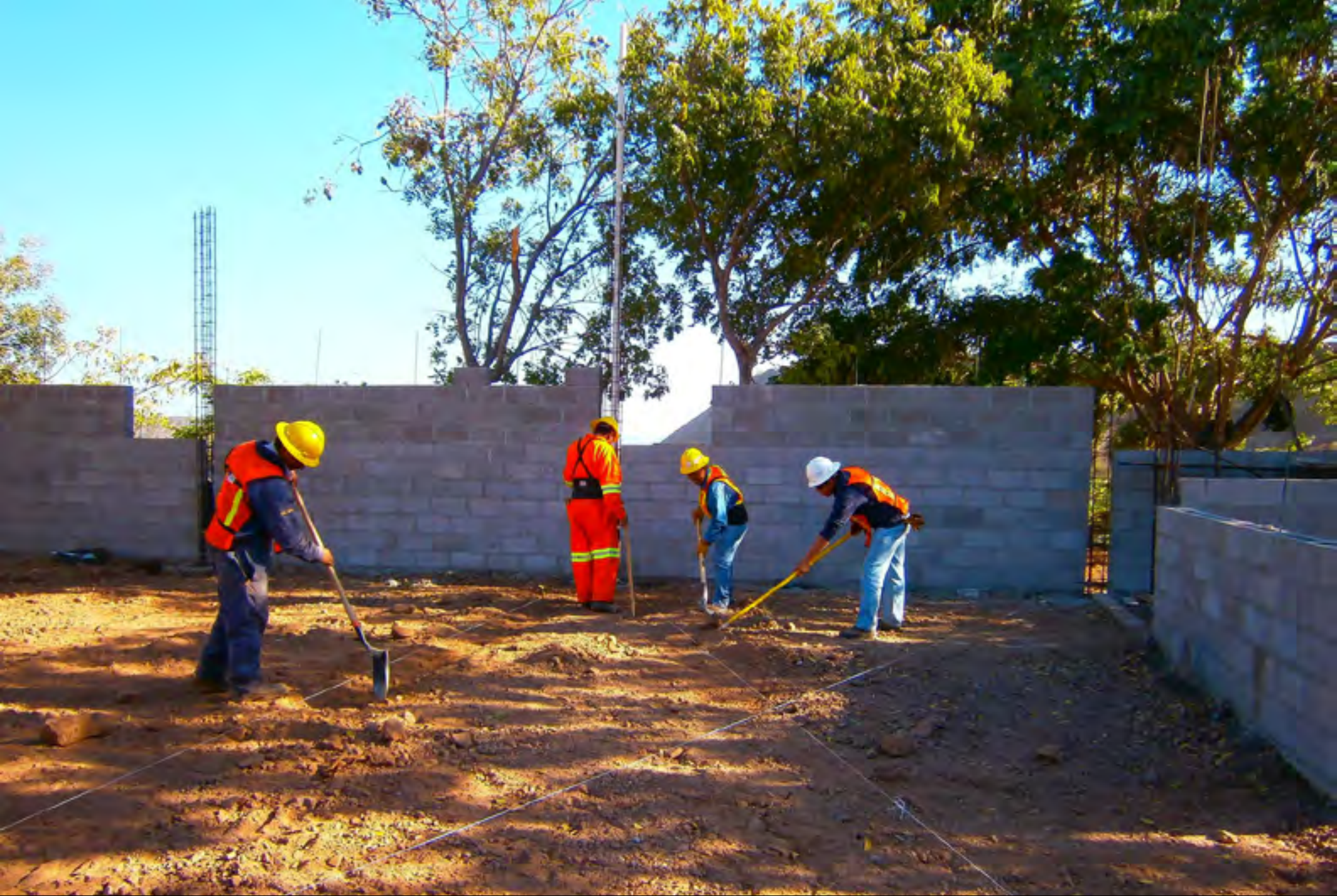
Walls for the new administration offices.
