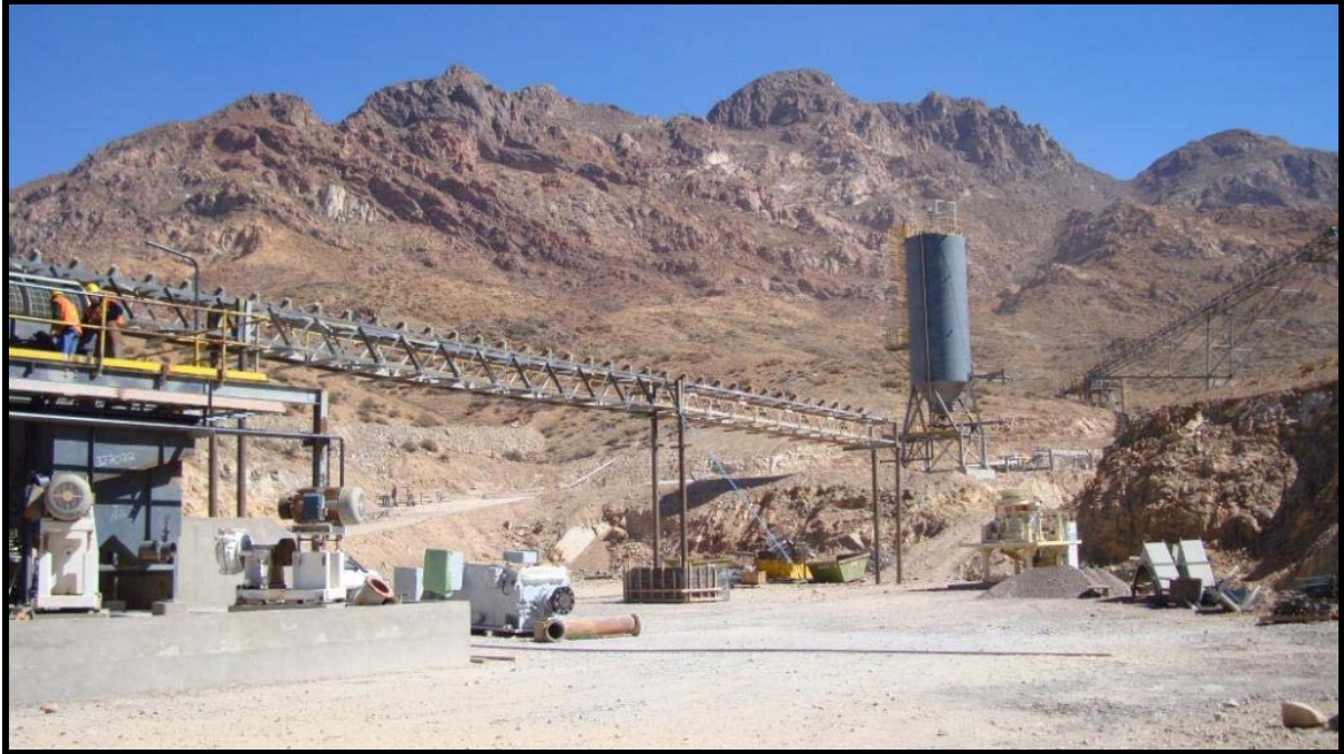
Mill feed conveyor with lime silo in background.
