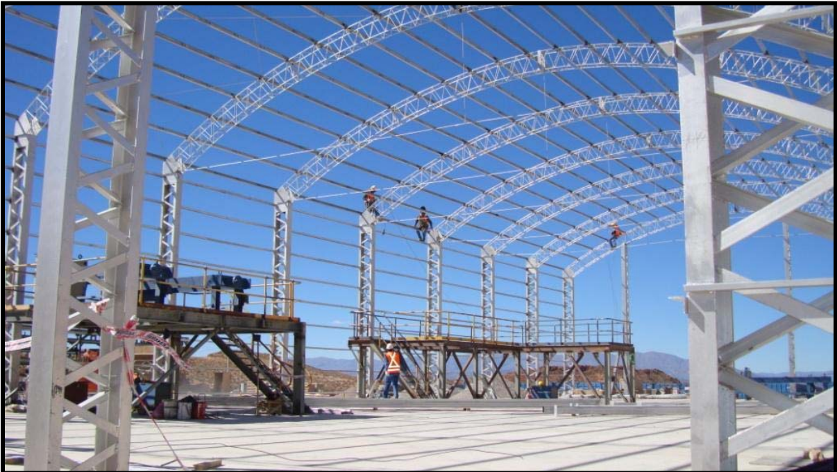
Merrill Crowe and refinery building under construction.
