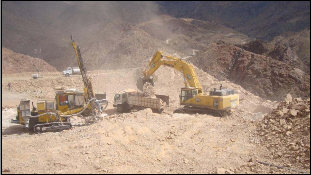
Kamila open cut pre-strip.
