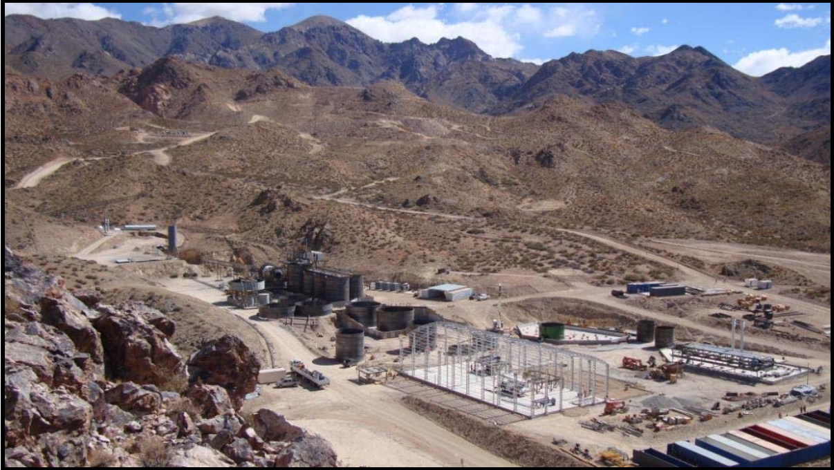
Casposo metallurgical plant lay out looking northwest with Merrill Crowe and tailings treatment area in the foreground, McKinnons plant in the middle and the crushing area to the left in the back ground.
