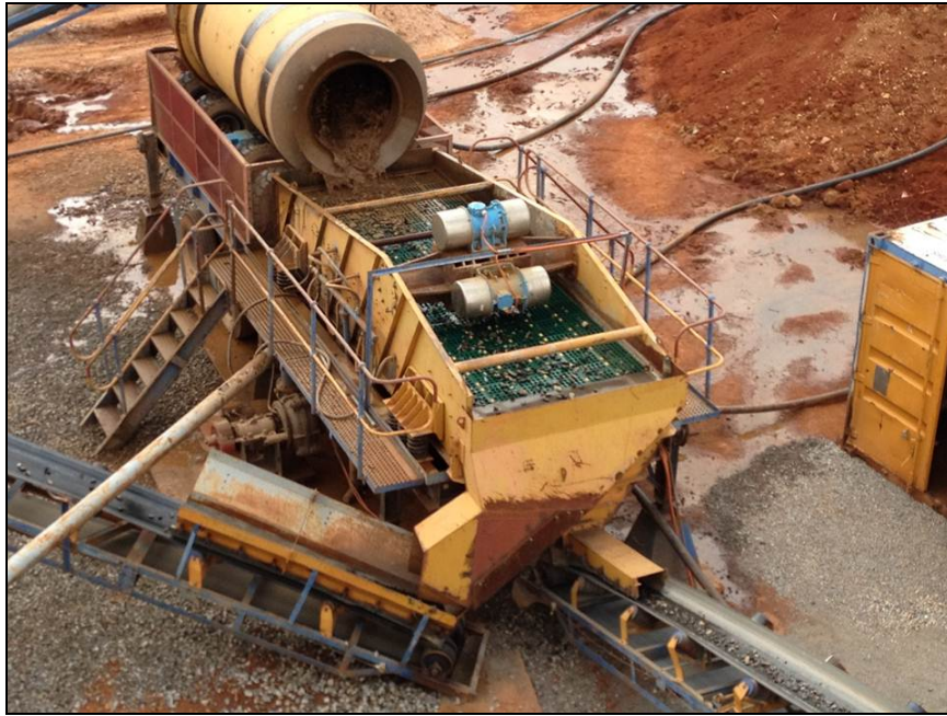
Photo 2: Pre-Production: Scubber unit with generator to the right, and conveyor to the DMS module in fore-ground.
