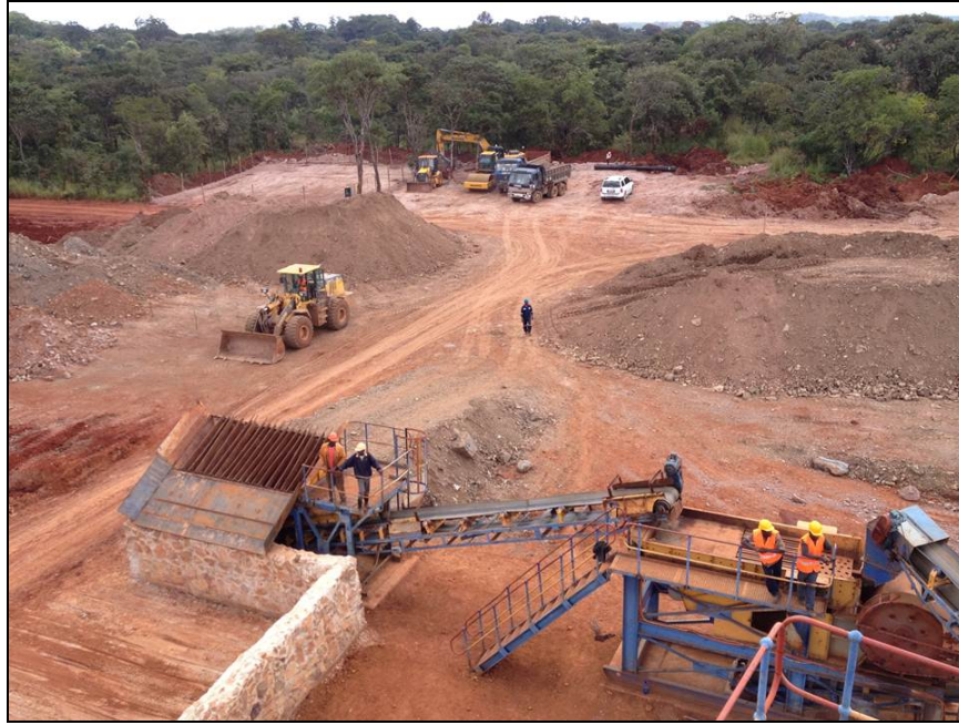
Photo 1: Pre-Production: ROM pad with feed bin and primary crusher in fore-ground.
