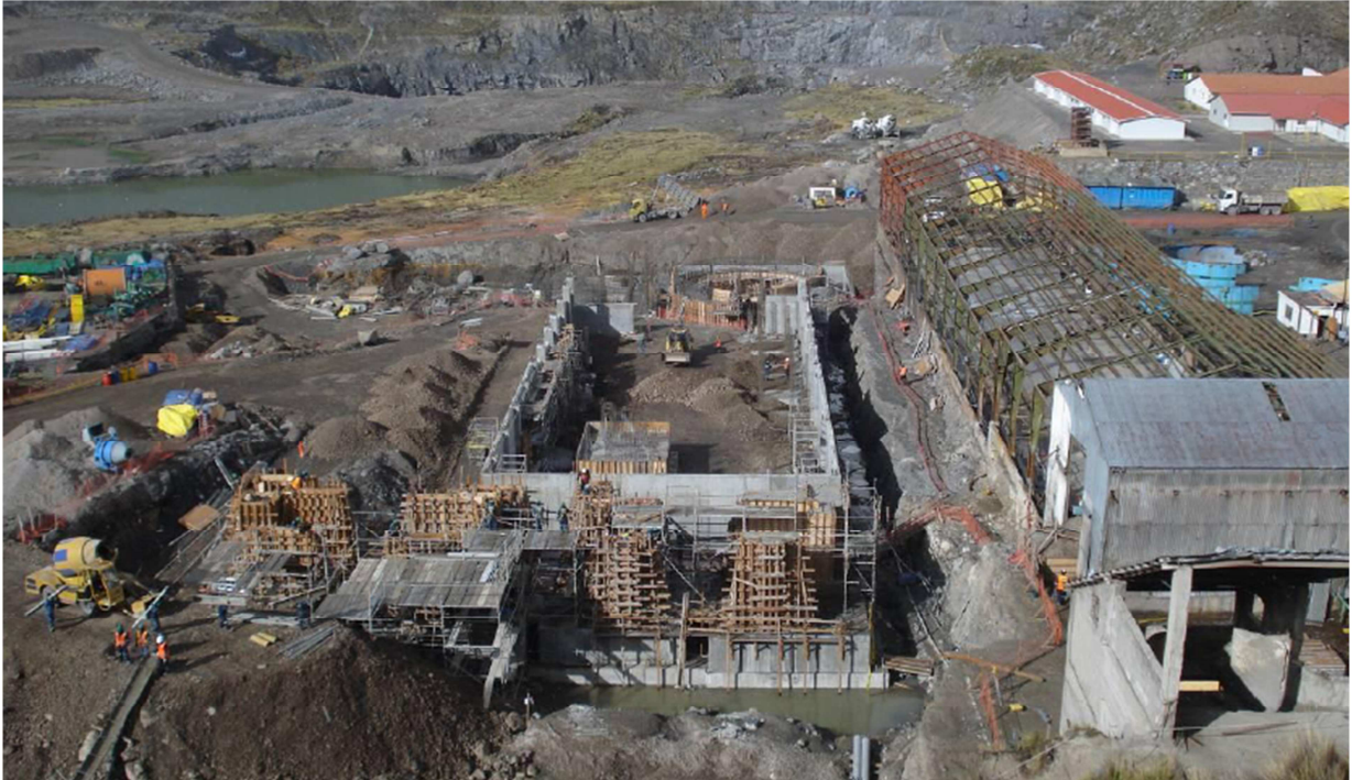
Figure 1: Construction of the Santander Mill and concentrate production buildings
