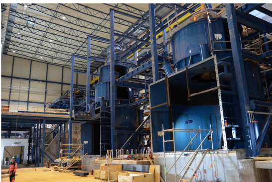
First sections of a Metso Vertimill capable of handling feed sizes up to 6 mm and grinding to a product less than 20 microns.
