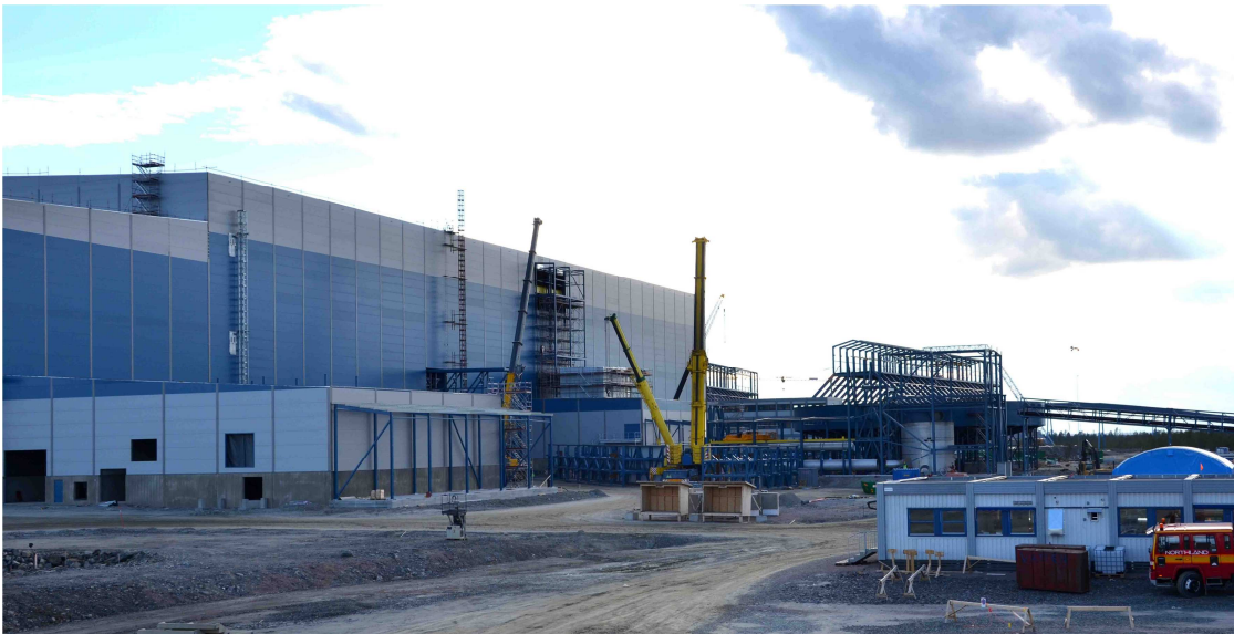
At the process plant in Kaunisvaara, work is currently focused on installation of crushers, mills, magnetic separators and electrical works. Adjacent to this building, work is ongoing to build the analytical and testing laboratory which will ensure that the product delivered to customer contains the high-quality magnetite that customers are expecting.
