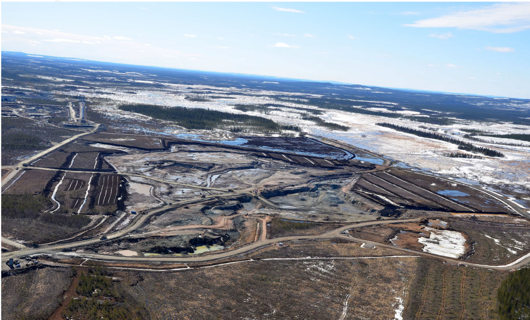
An aerial view of the Tapuli mine, where the removal of the overburden proceeding according to schedule. Activities are ramping up to start the production in Q4 2012.
