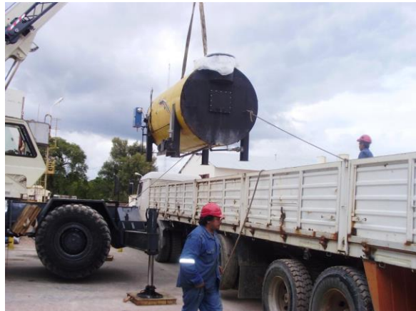
Boiler being loaded for relocation
