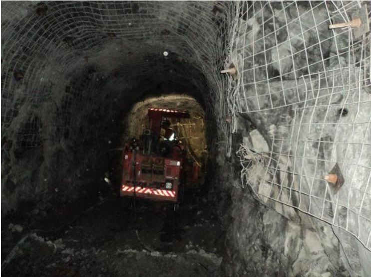
Figure 4: Jumbo Drilling at the 244-metre Level Exploration Drift
