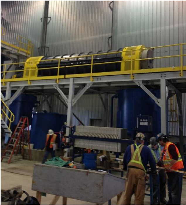
Figure 2: Elution Plant Construction
