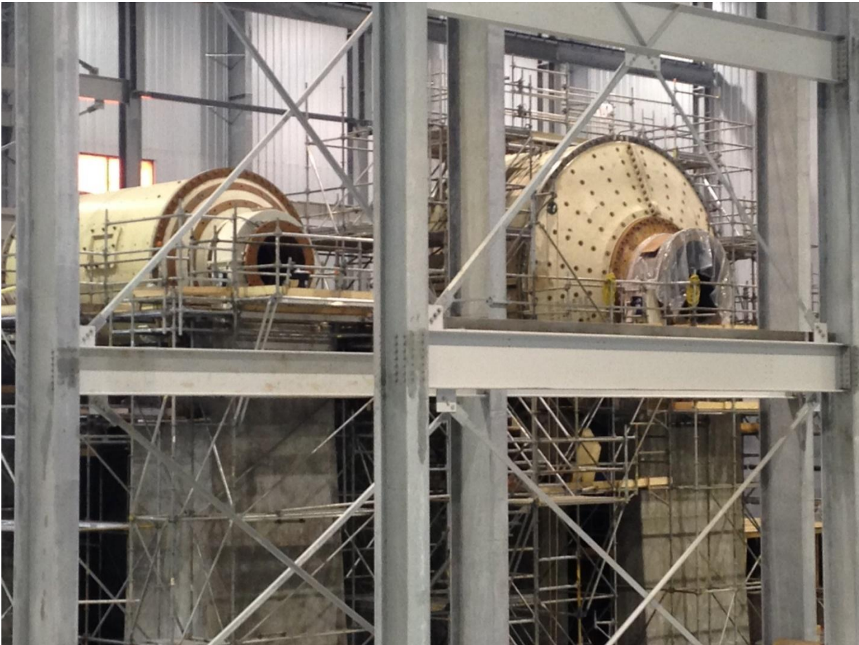
Figure 2: SAG and Ball Mill Installations
