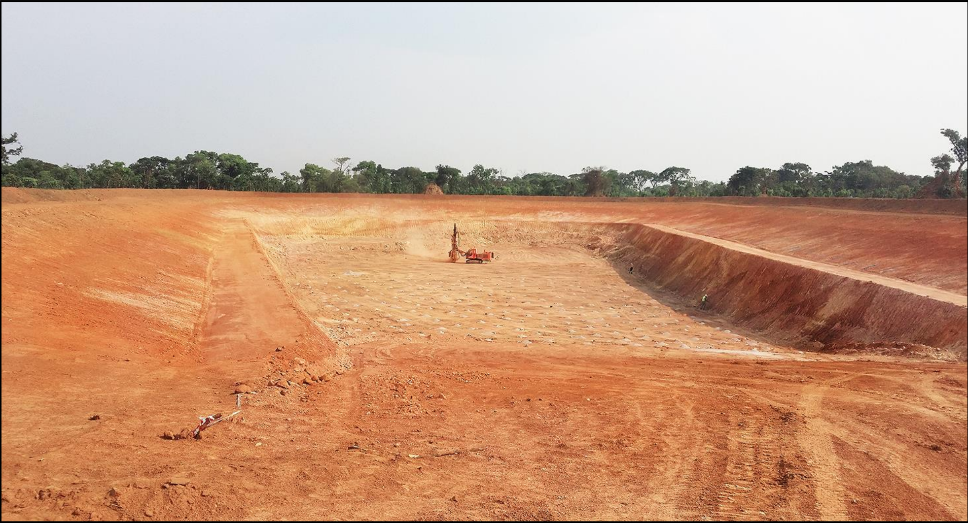
Figure 3: Blasting at box-cut site, September 20, 2014.
