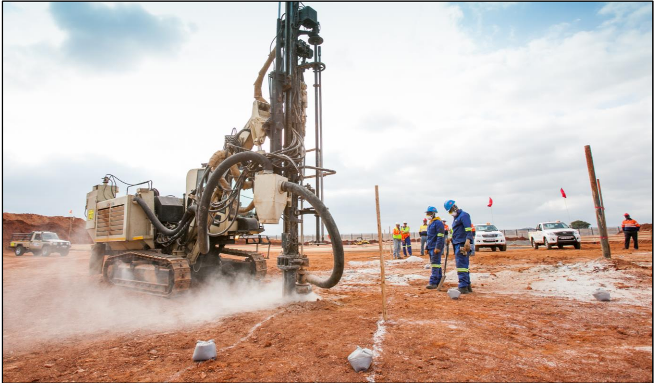
Photo 3: Holes being drilled in preparation for first blast at the box cut.
