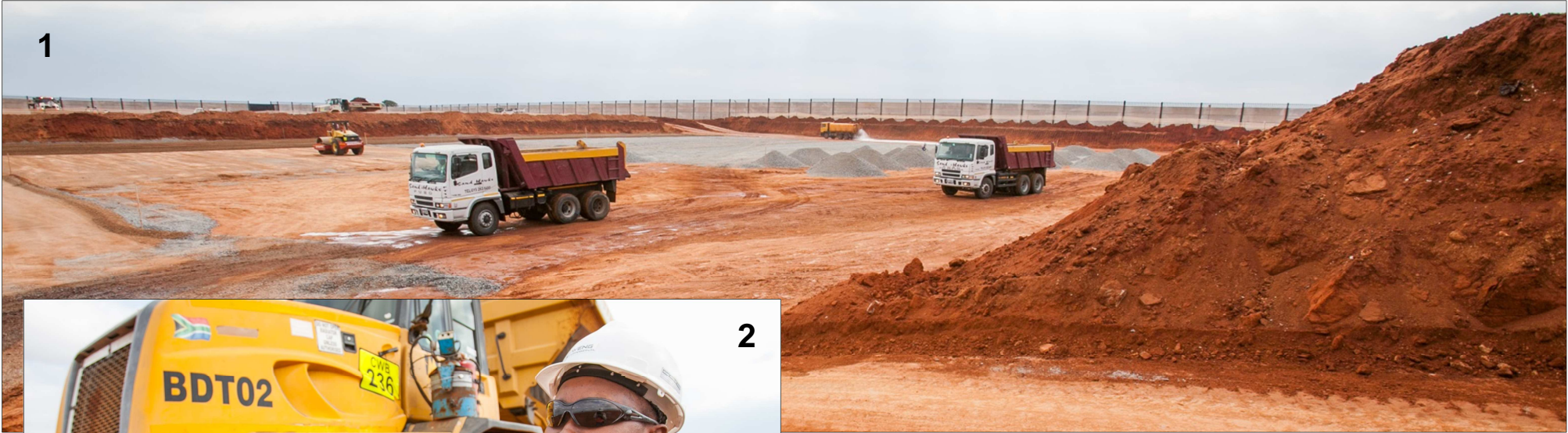
Photos 1 to 3: Earthworks for sinking of Shaft No. 1.
