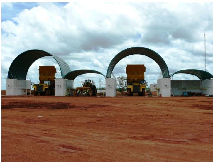
Truck workshop and service area
