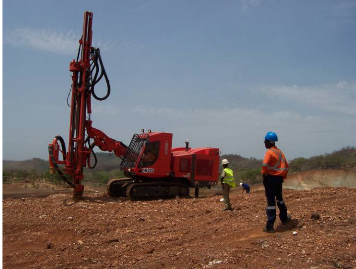
Pantera drill rig positioned on the ore zone with open pit edge in background
