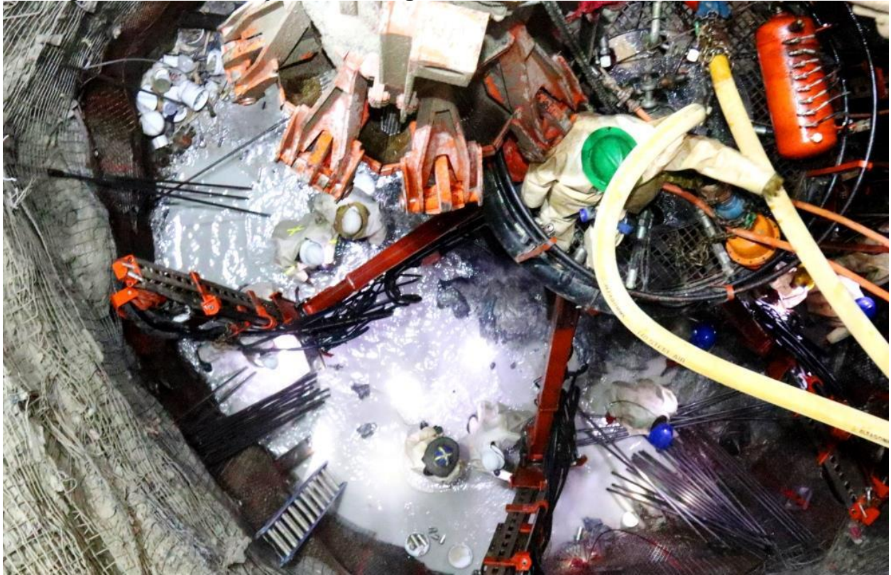
Drilling with a six-boom jumbo drill rig at the bottom of Shaft 1.
