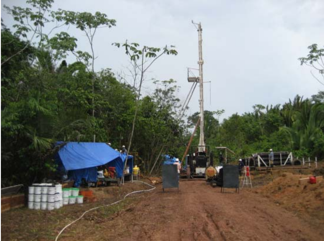
Diamond drill set-up, Autazes area, Brazil Potash project.
