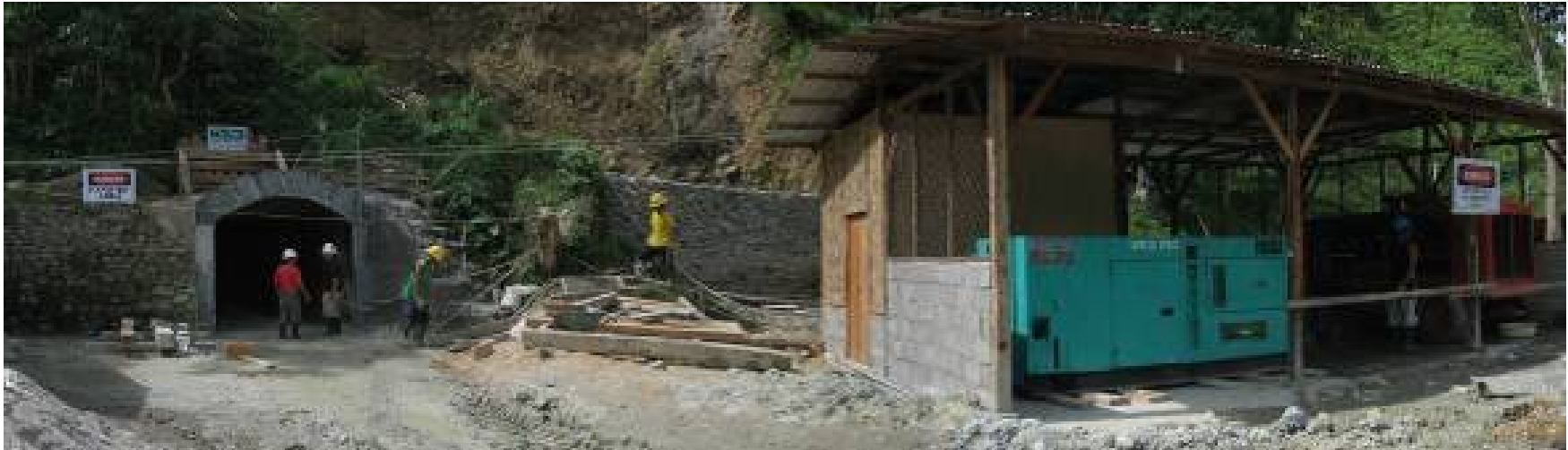
Above is the new Mafoko Portal (left) being constructed to enable mechanized operations and the powerhouse at the T'Boli gold-silver project.
