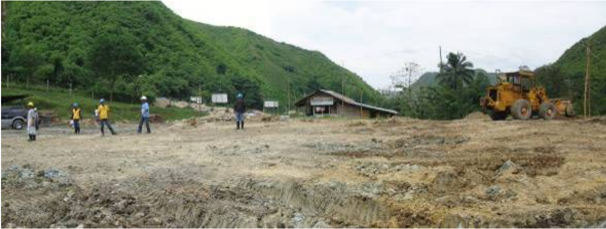
Above: the area outside the Mafoko Portal being prepared for a possible future plant.
