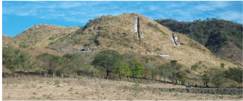
Trenching underway on the Central Breccia during 2012.
