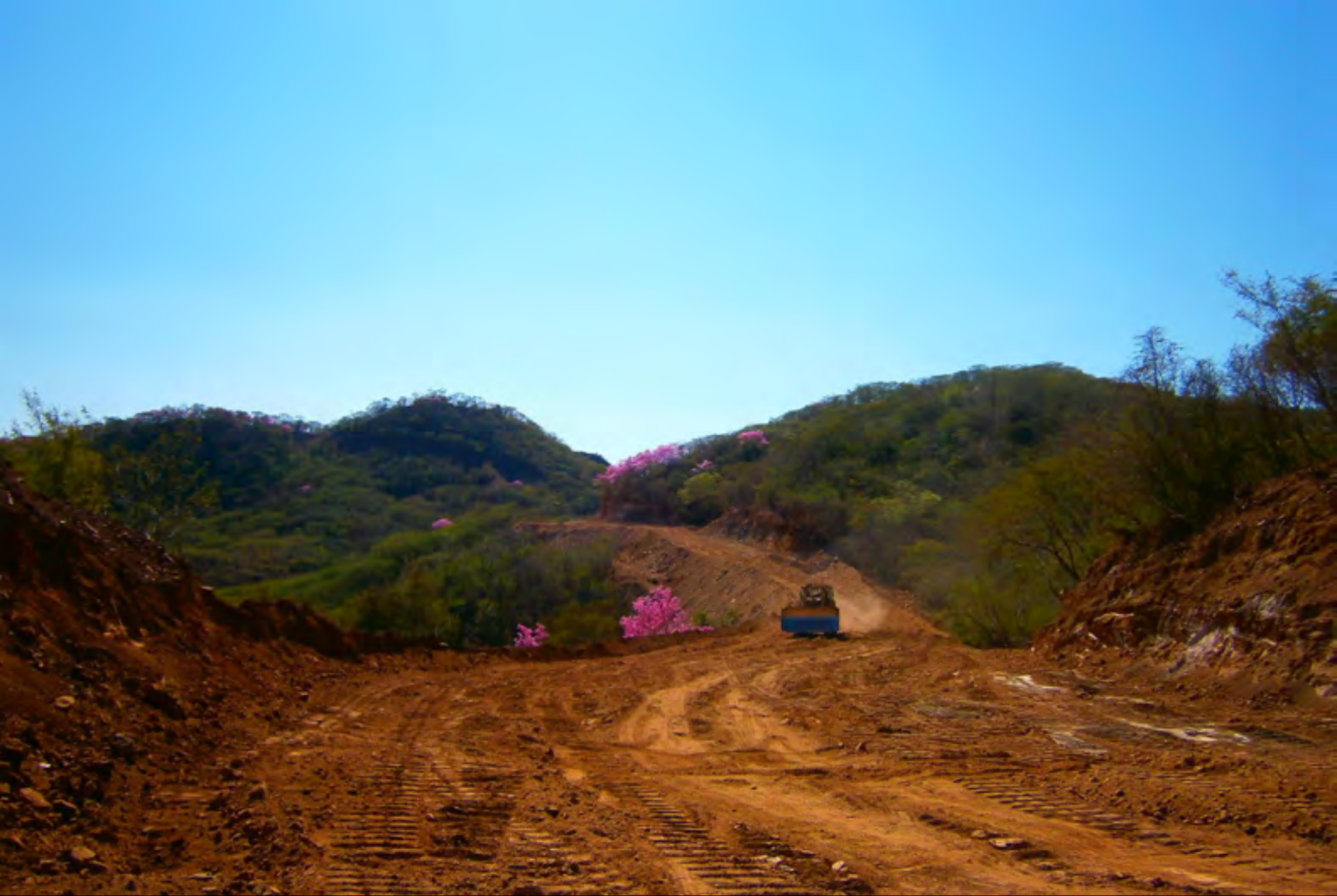
Haul road to the Sargrado Corazon deposit nears completion.
