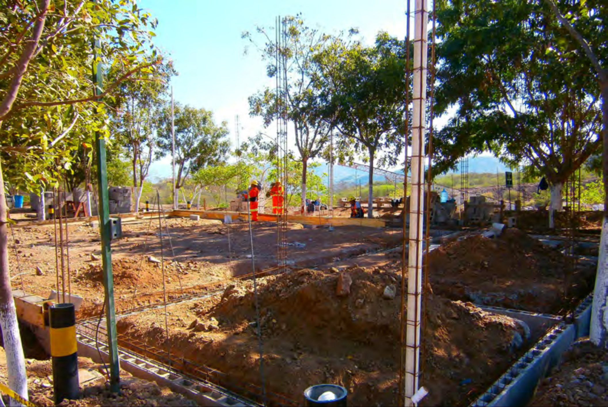
Foundation for new administrative building.
