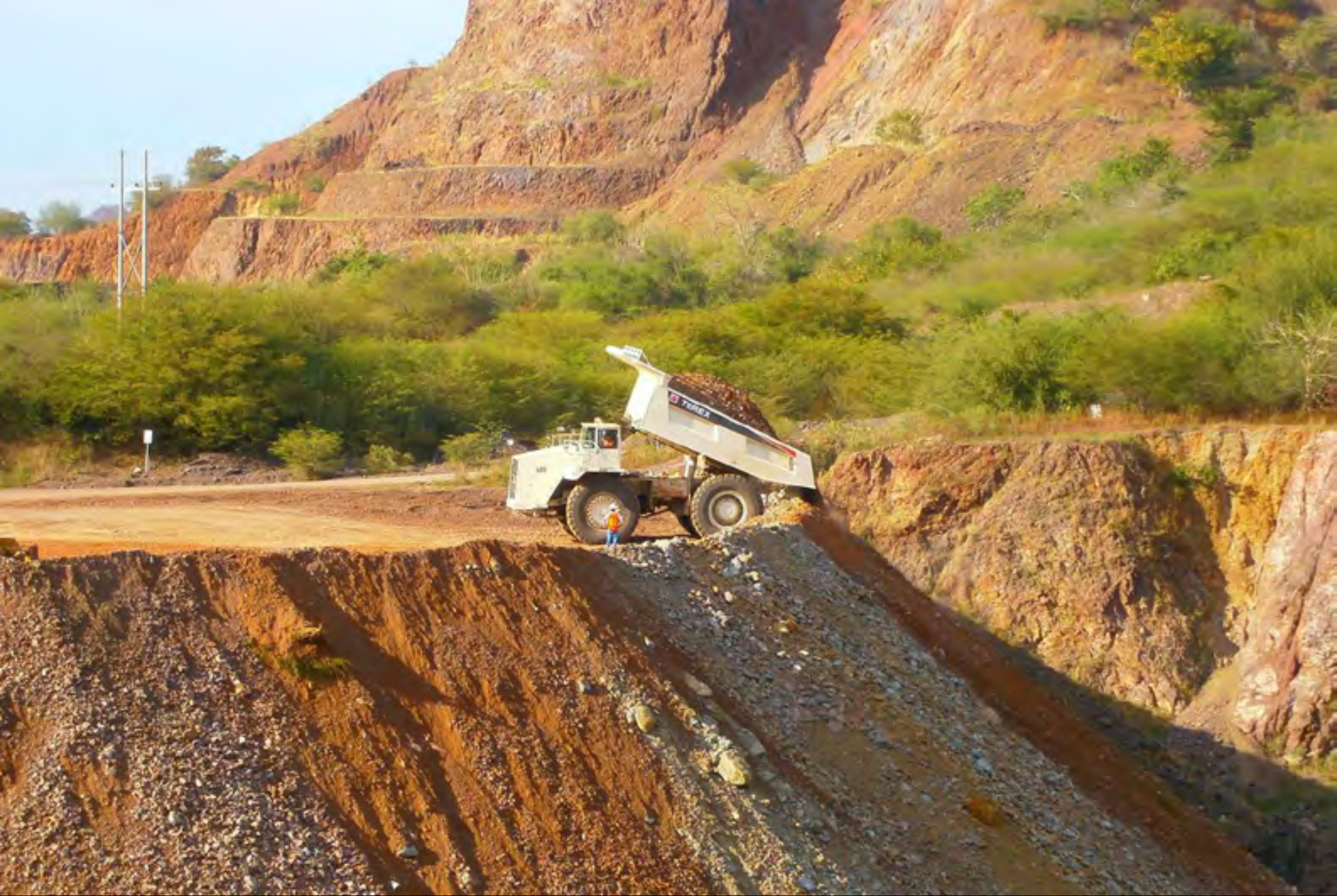
Back filling the previously mined open pit.
