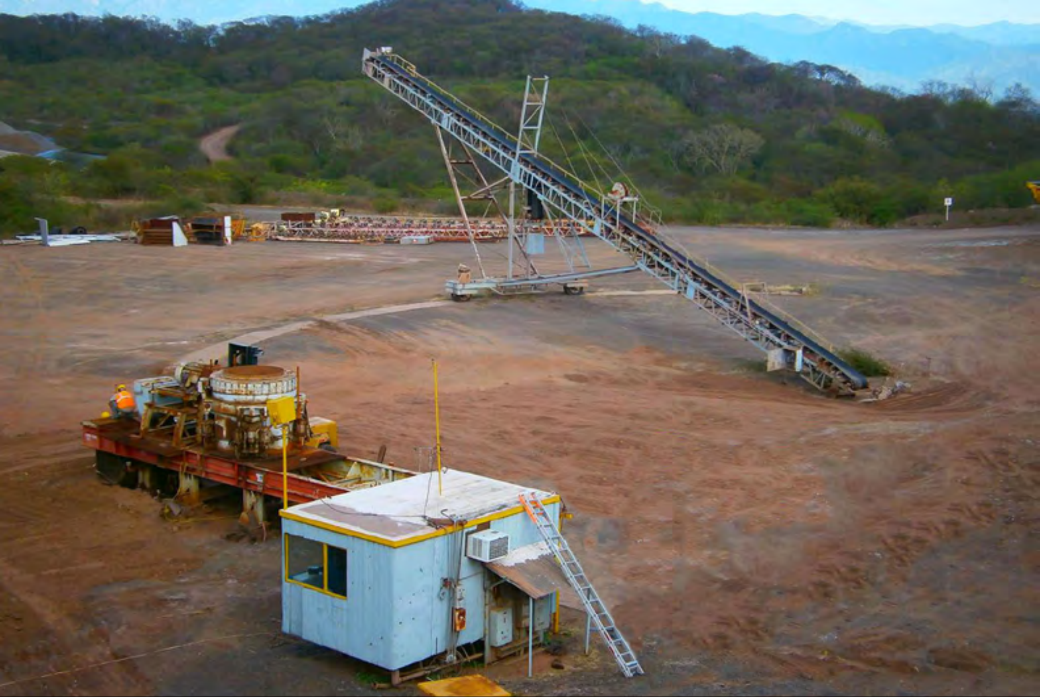
Decommissioning of the previous crushing plant.
