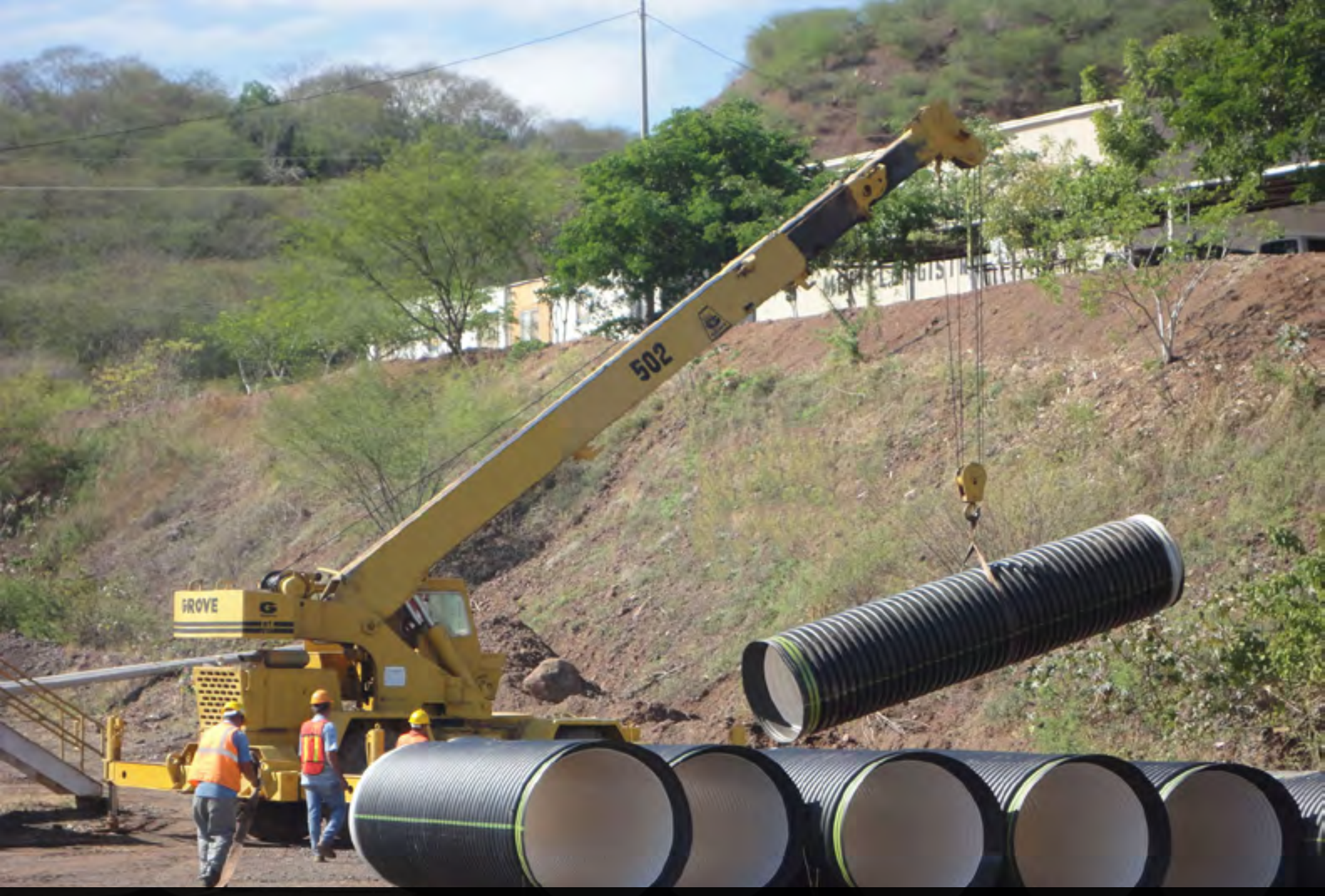
Culverts being moved into place around the crushing plant.
