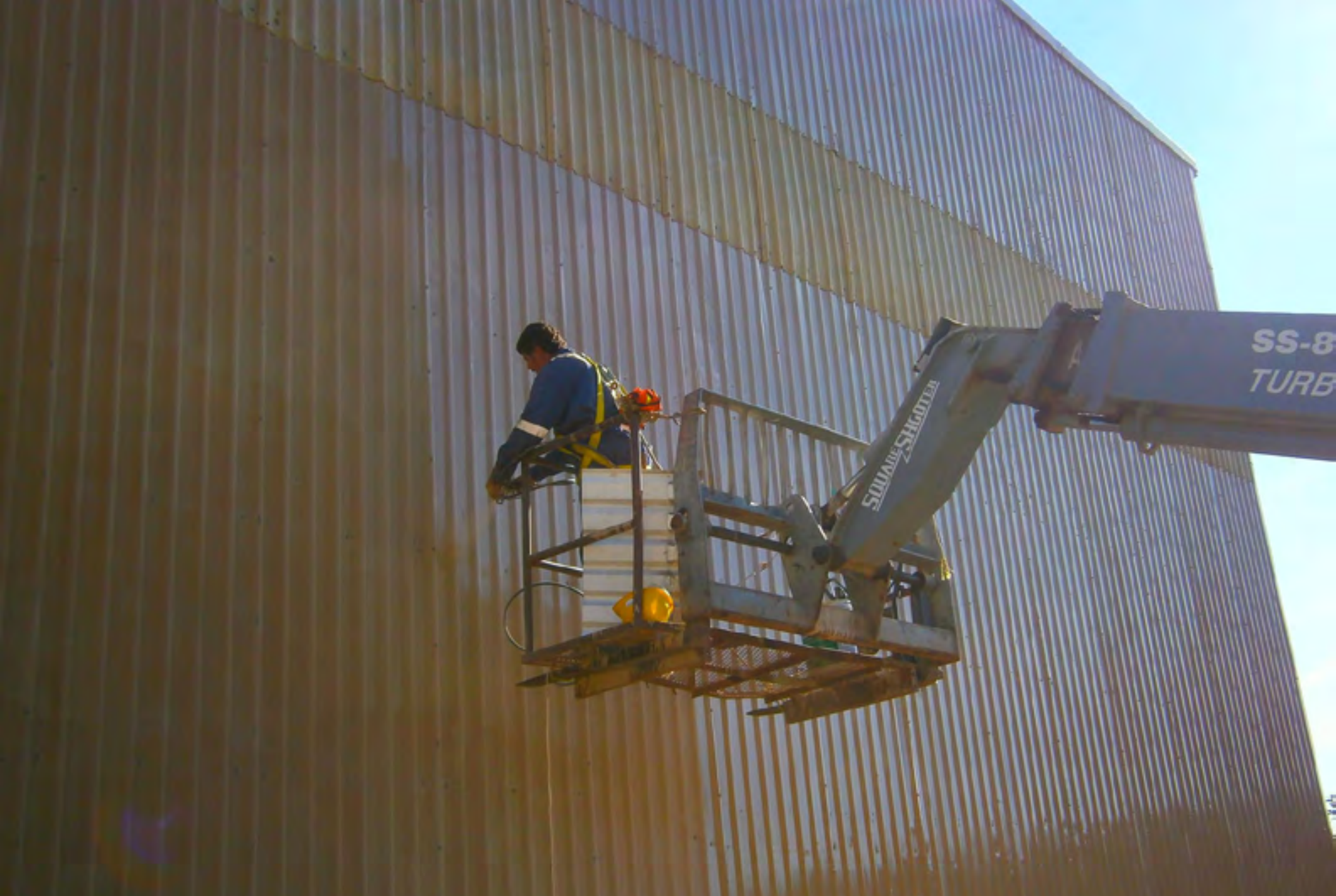
Painting existing buildings.
