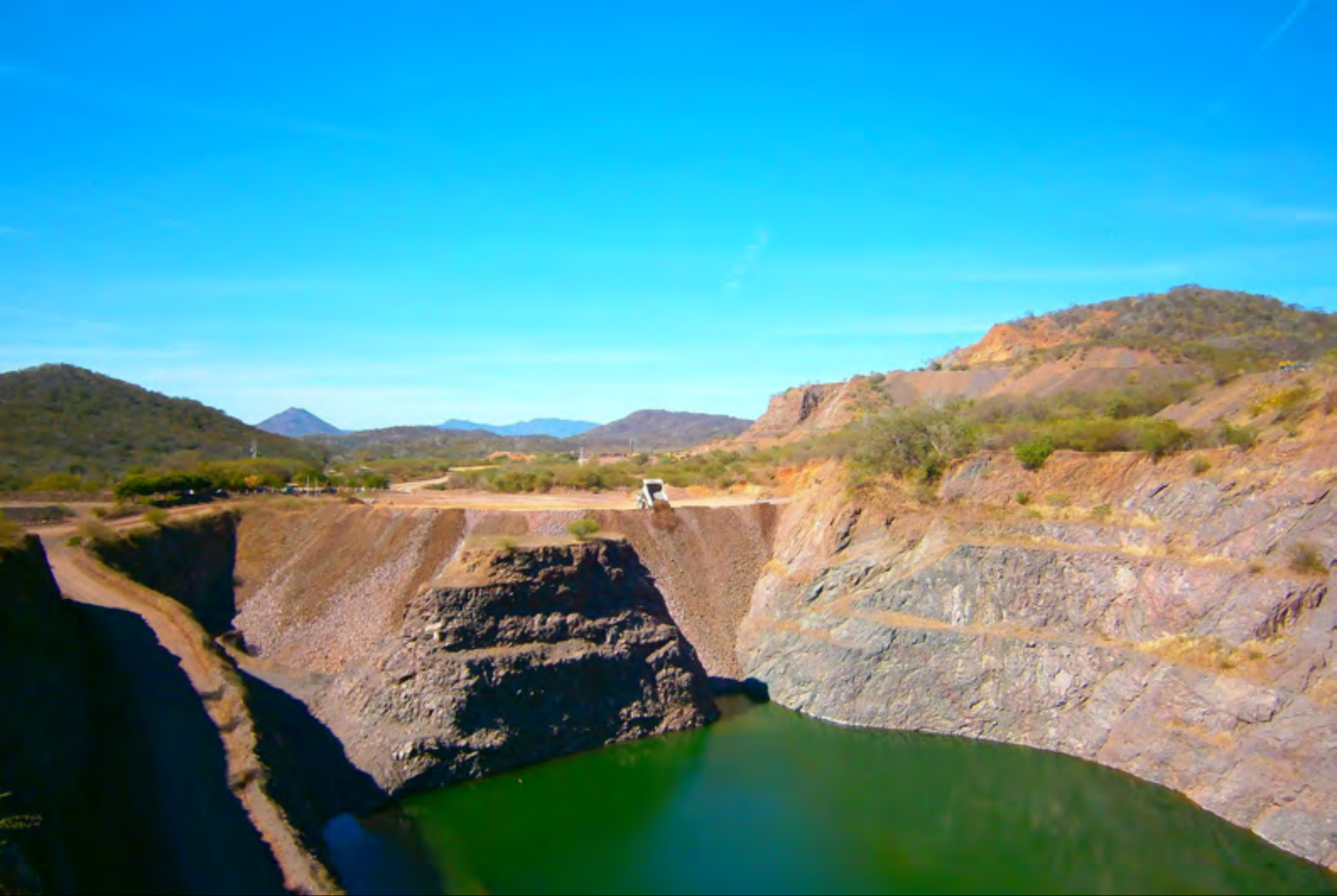
Pre-stripping (background) and backfilling (foreground).
