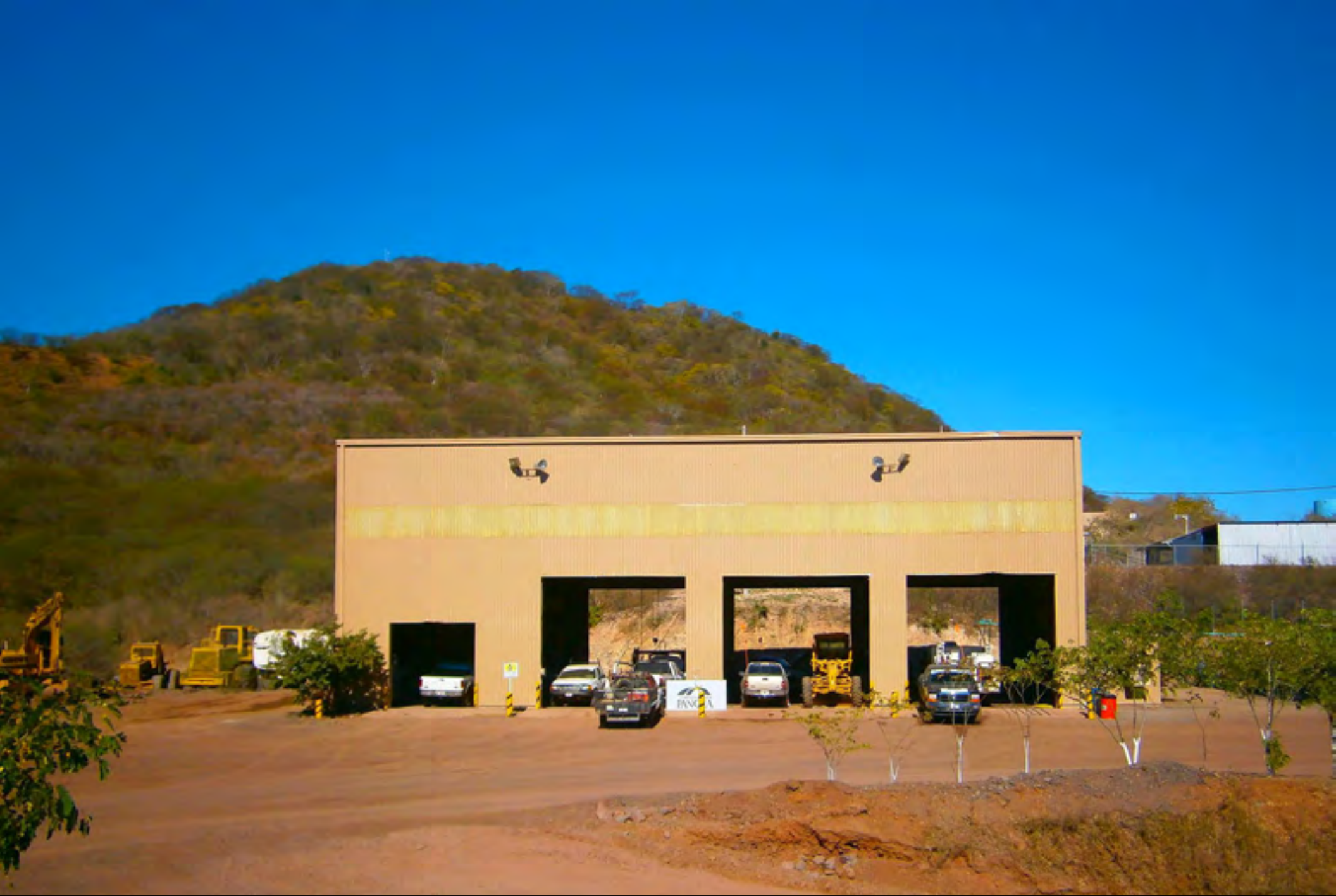
Painting of maintenance shop completed.
