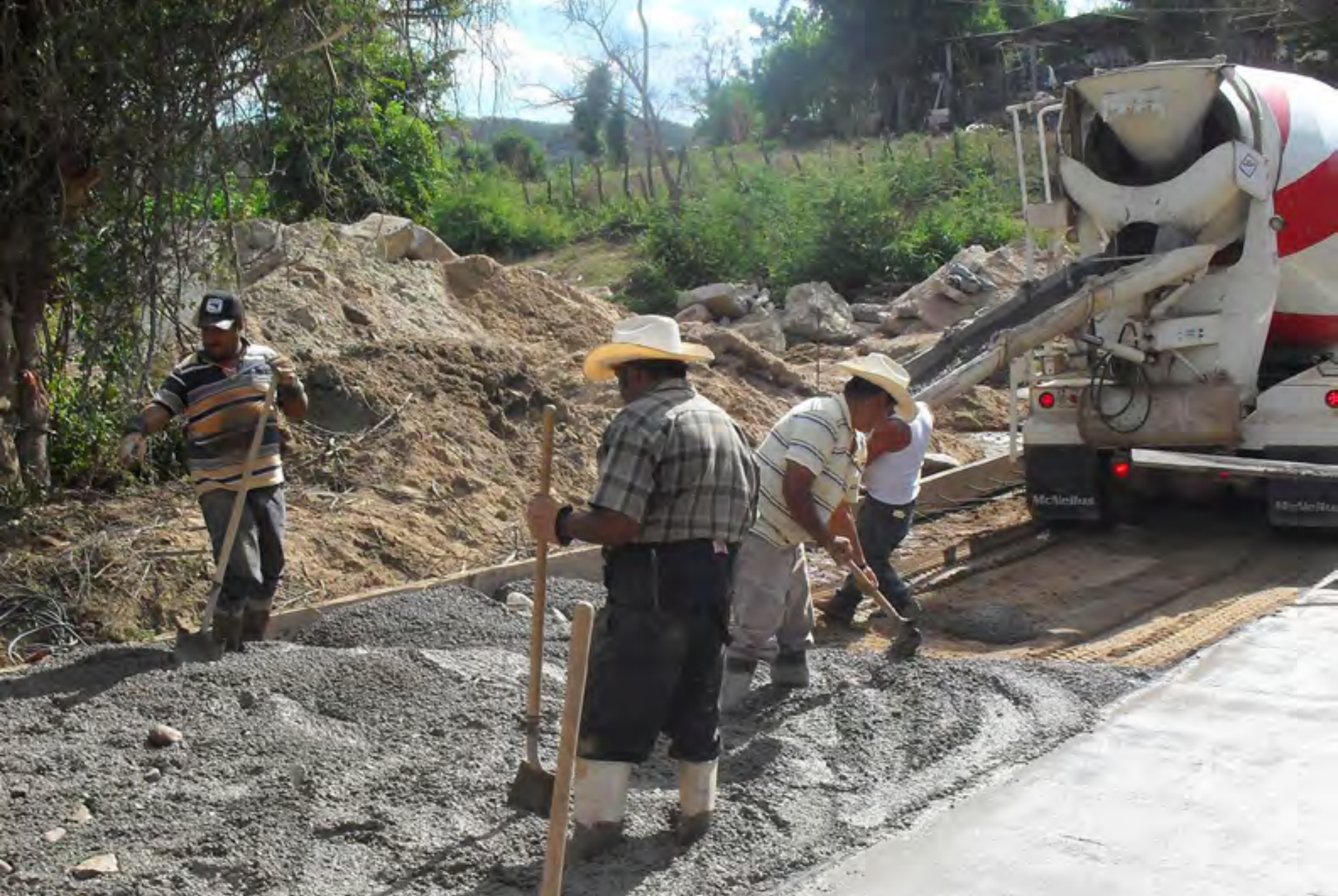
Bridge construction along the haul road between the El Gallo and Palmarito deposits.
