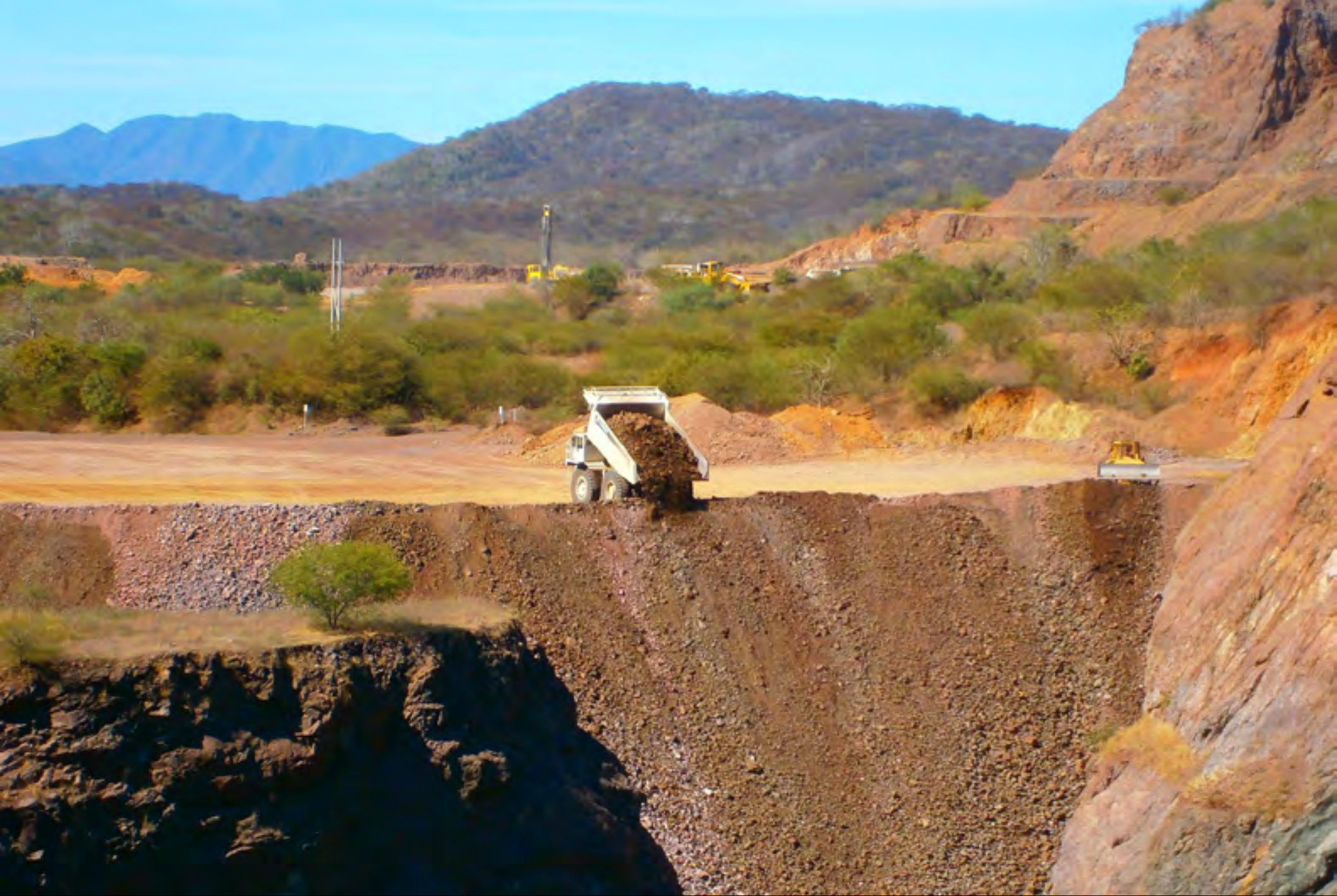
Pre-stripping (background) and backfilling (foreground).
