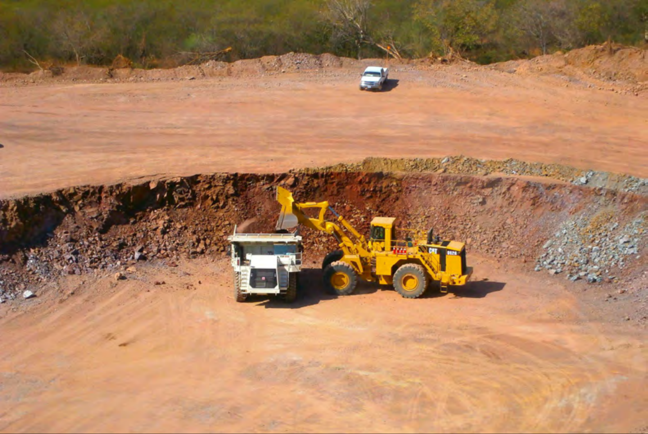
Pre-stripping in Samanegio open pit.
